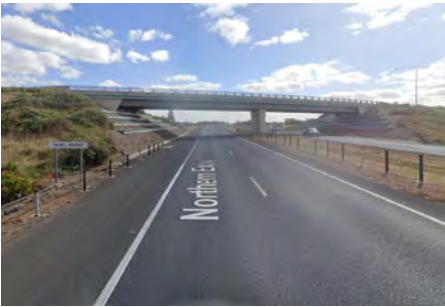
Below: Penfield Rd overpass (Hamel Bridge) on North-South Motorway - 5.3m clearance.
