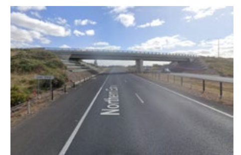
Below: Penfield Rd overpass (Hamel Bridge) on North-South Motorway - 5.3m clearance.
