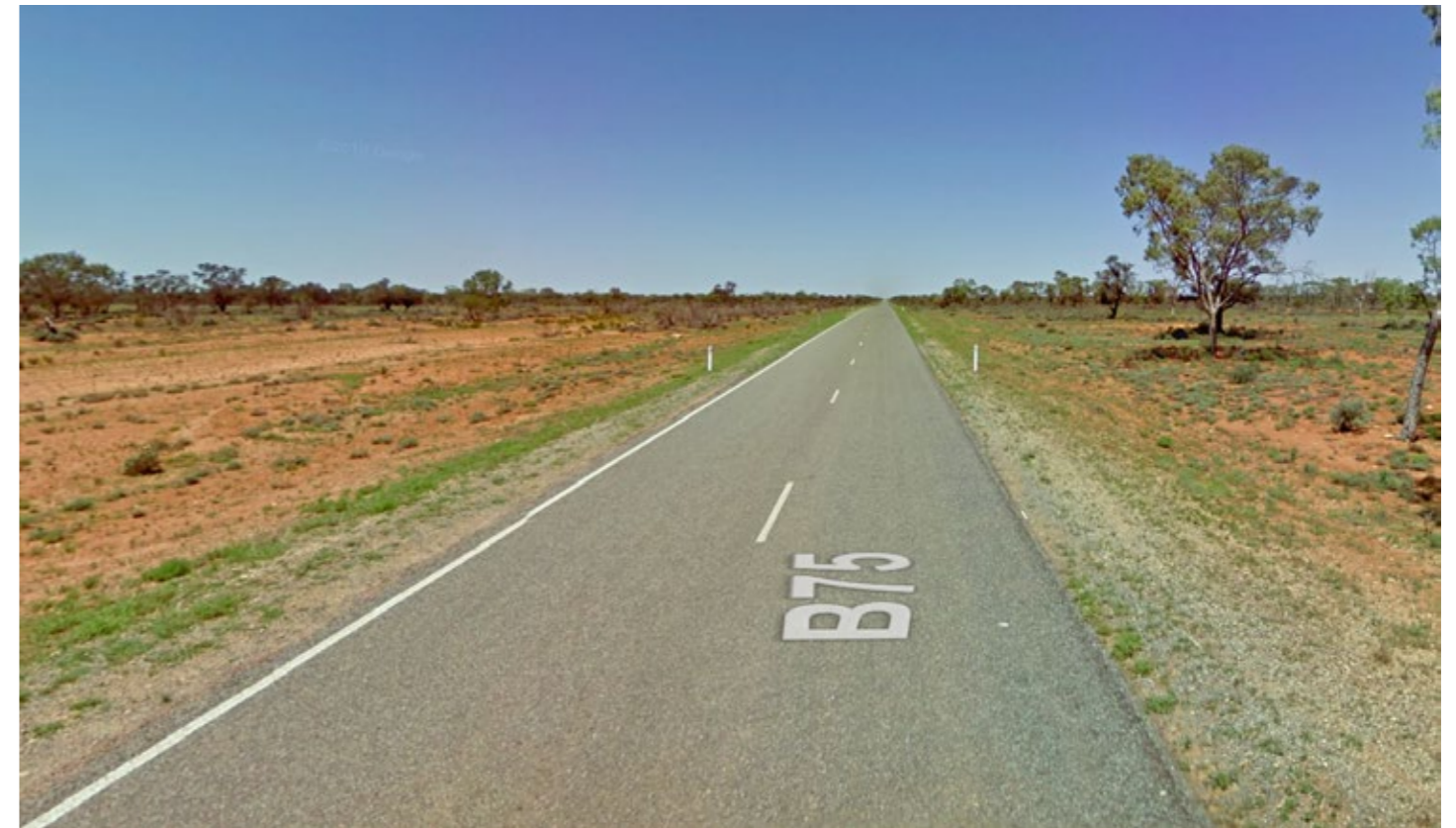
Above: Typical construction of Cobb Hwy with minimal shoulder.
