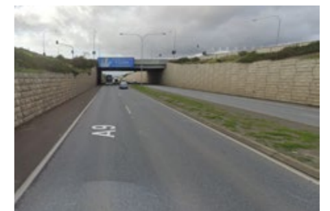
Above: Hanson Rd overpass of Port River Expressway - 6.0m clearance.
