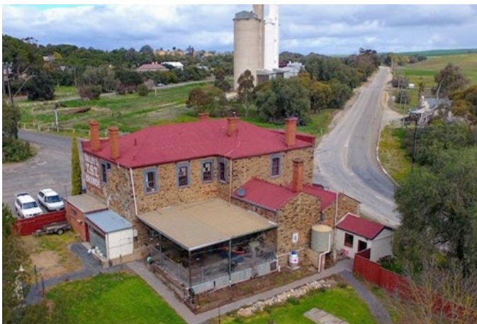
PHOTOGRAPH 3-6 CURRENT BON ACCORD HOTEL WITH REAR BLUESTONE EXTERIOR, LOOKING SOUTH-WEST (KEVIN EATTS)
