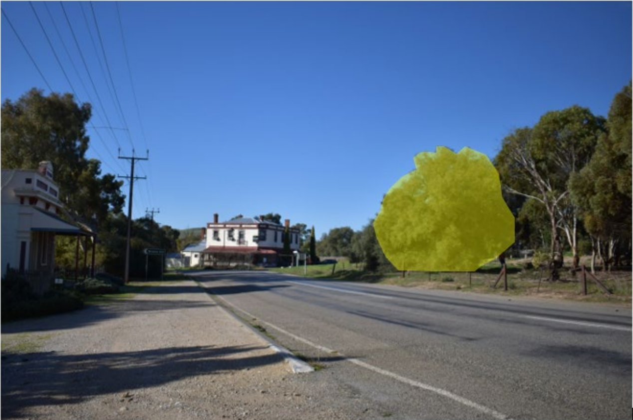
PHOTOGRAPH 4-1 PINCH POINT 08, LOOKING NORTH-EAST ON COPPERHOUSE STREET TOWARDS THE BON ACCORD HOTEL. THE TREE SUBJECT TO REMOVAL IS OUTLINED IN YELLOW (ERM, 2023)
