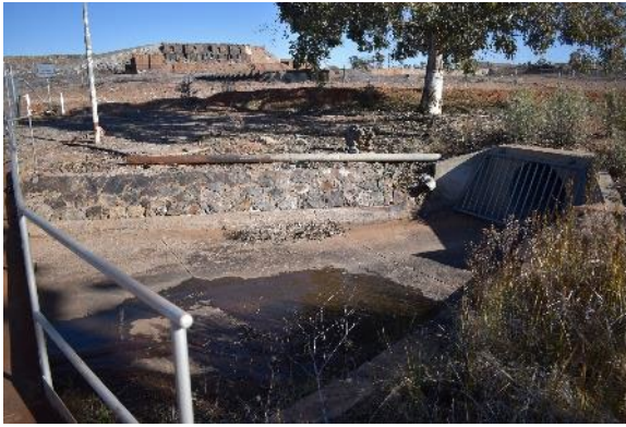
PHOTOGRAPH 4-1 VIEW SOUTH OF THE DRAINAGE CHANNEL TO THE SOUTH OF THE PROPOSED ACTIVITY AREAS (ERM 2023)
