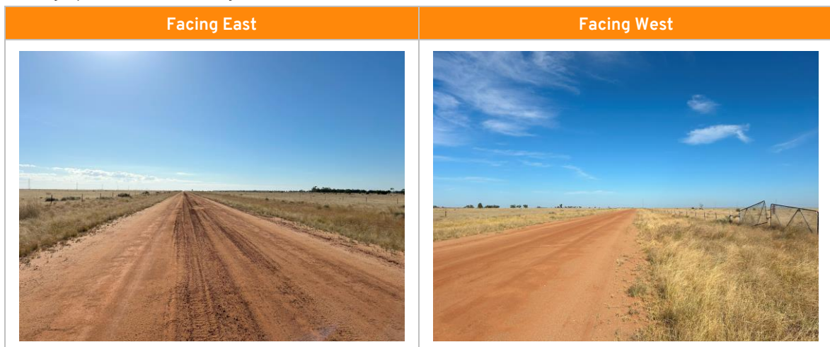
Photograph 2: West Burrabogie Road
