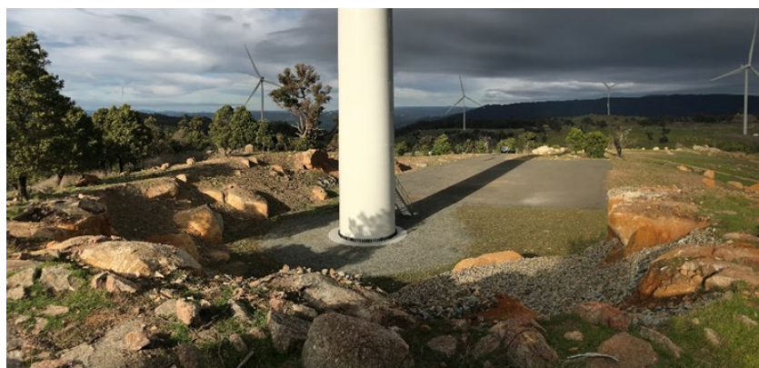
FIGURE 3-5 TYPICAL HARDSTAND AREA
