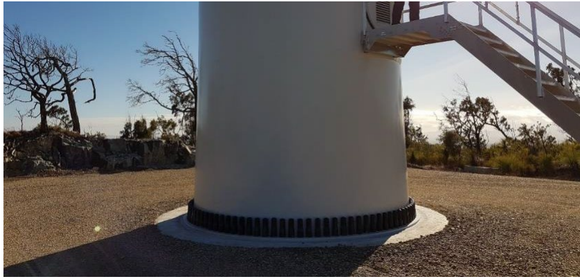
FIGURE 3-4 TYPICAL WTG FOUNDATION POST-CONSTRUCTION
