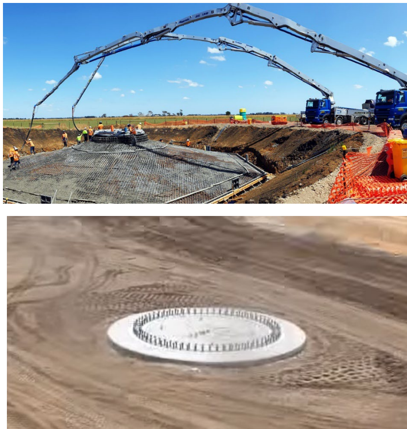
FIGURE 3-3 TYPICAL WTG FOUNDATION UNDER CONSTRUCTION
