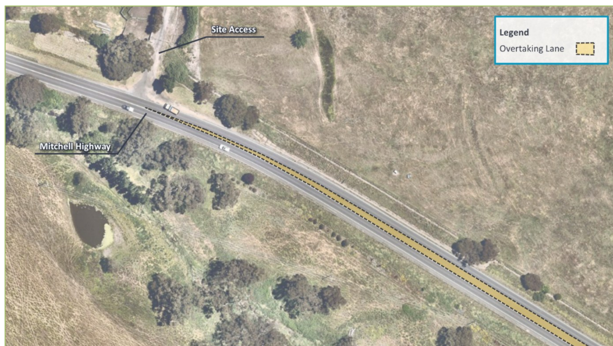
Figure 4 Overtaking Lane on Mitchell Highway
