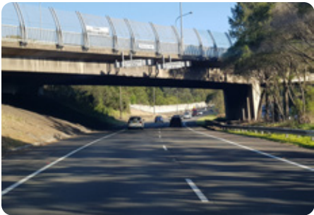
Below: Princes Hwy overpass of M1 Motorway - 5.3m clearance in right hand lane
