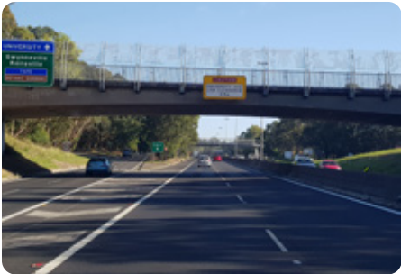
Above: University Avenue overpass of M1 Motorway - 5.2m clearance in left hand lane
