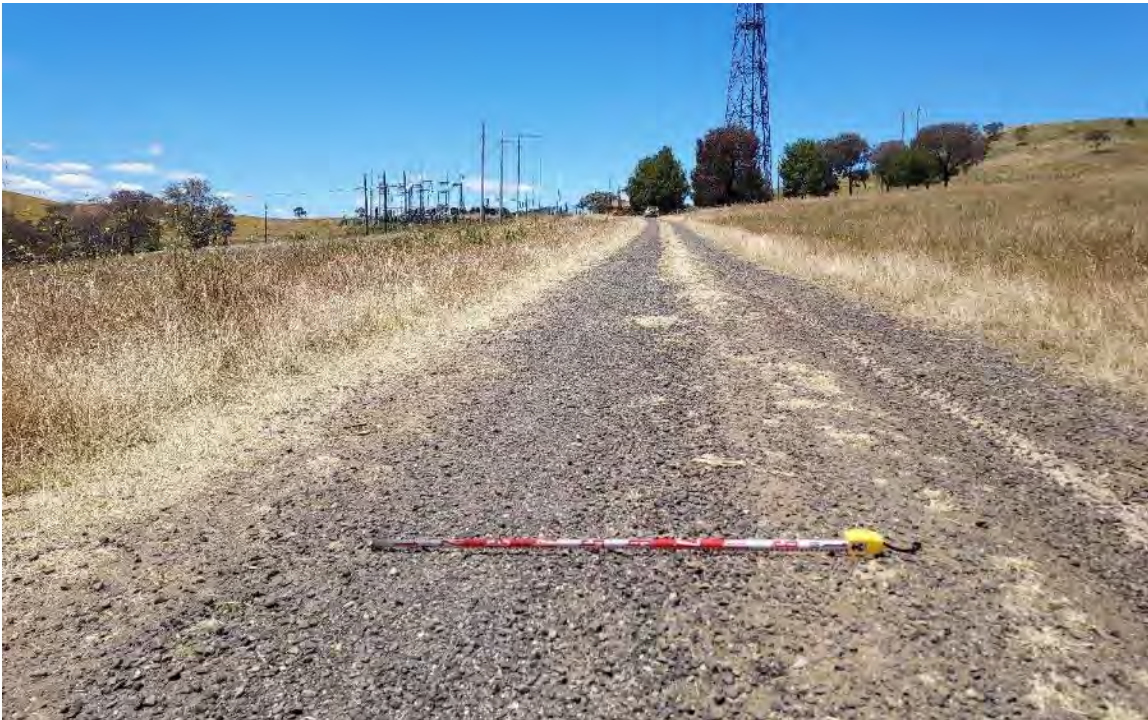
Figure 7.1 East-facing view of disturbed existing access road.
