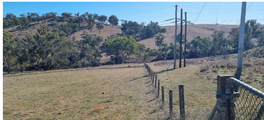
Figure 14-2 Transmission line infrastructure in the Transgrid Lot
