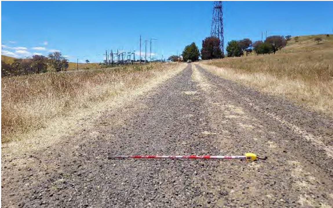
Figure 7.1 East-facing view of disturbed existing access road.
