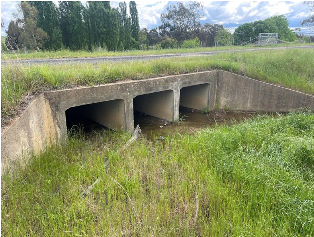
Photo B-3 Box culvert under access road to substation
