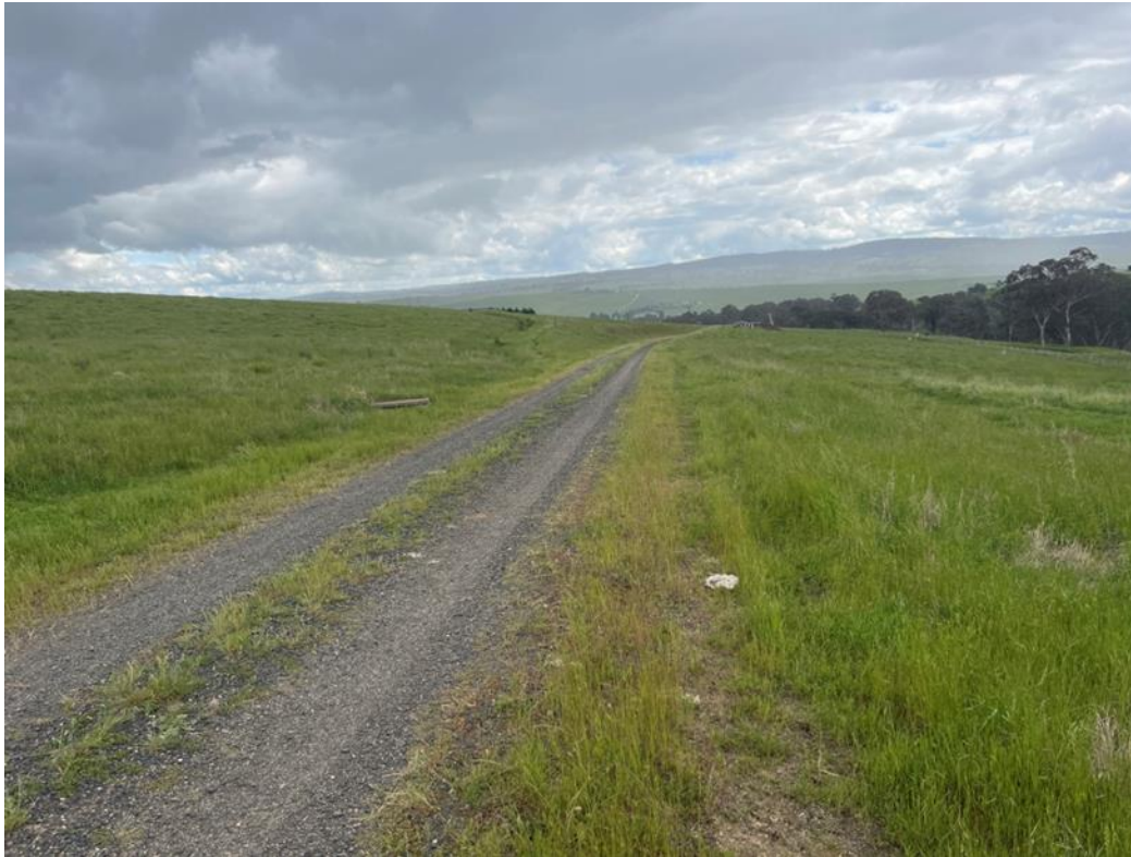
Photo B-6 Existing access road through subject land
