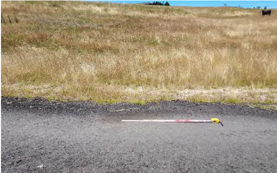
Figure 7.2 South facing view of disturbed access road adjacent to slope.
