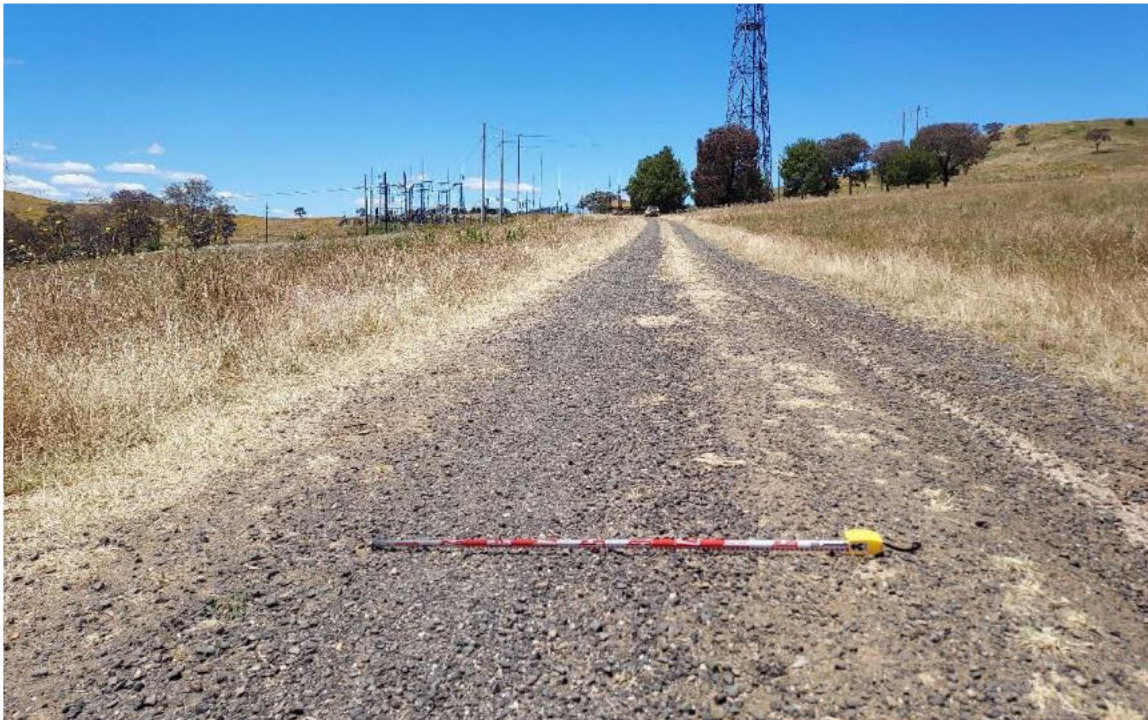
Figure 7.1 East facing view of disturbed existing access road.
