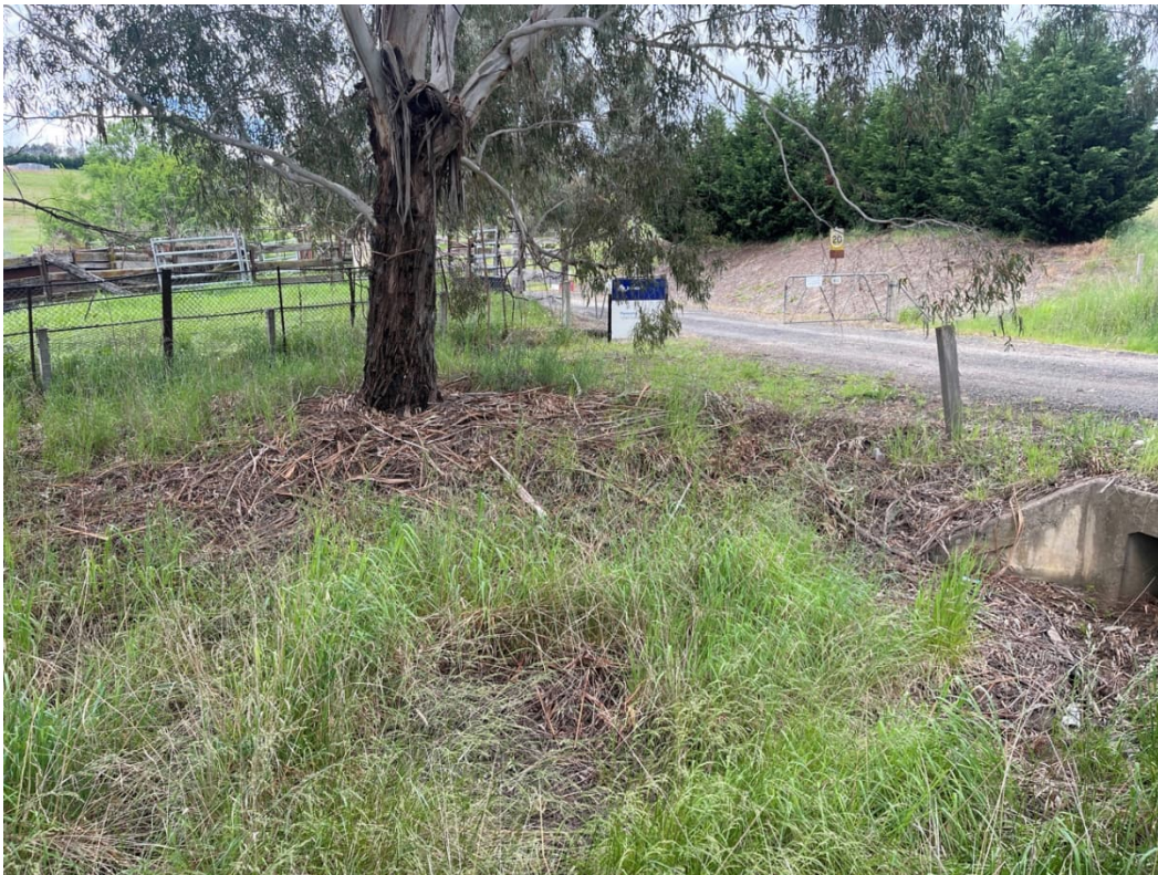
Photo 5 Culvert at subject land access road entry and Eucalyptus viminalis
