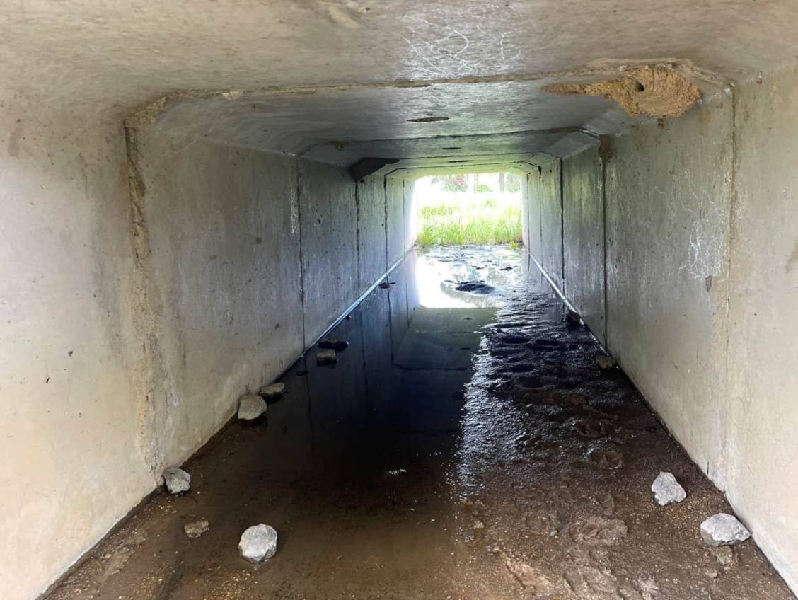
Photo 4 Culvert with mud nests along access road
