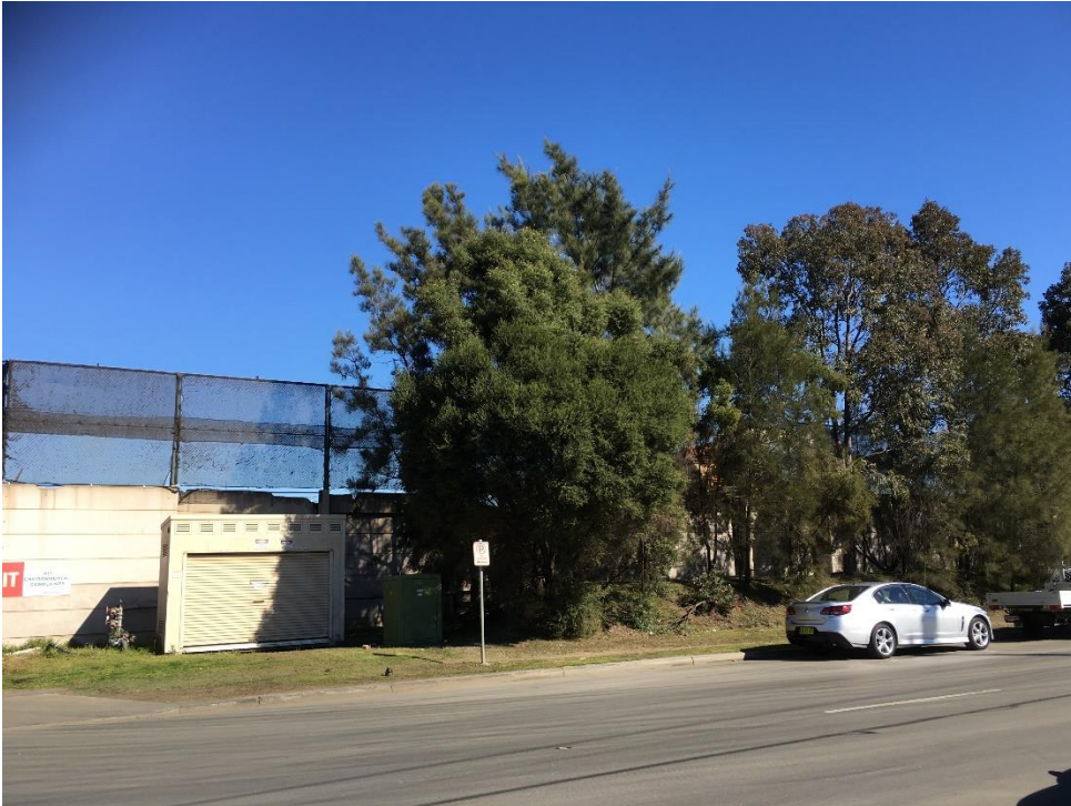
Photograph 1: View of site frontage to 45 Tattersall Road
