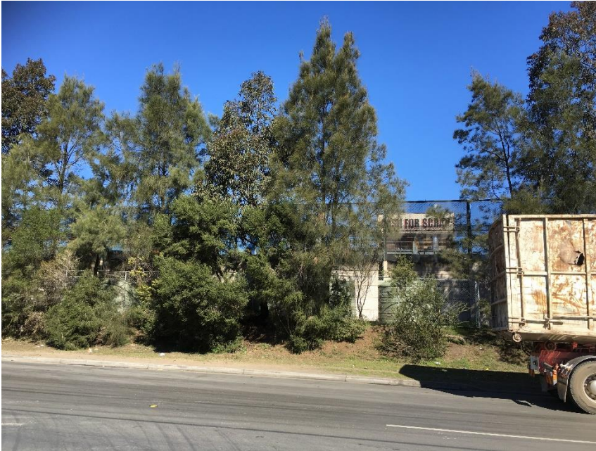
Photograph 2: View of site frontage to 45 Tattersall Road
