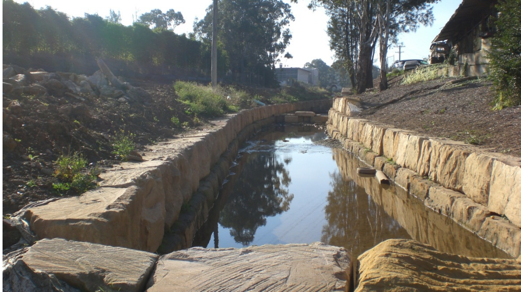
Photograph 6.3 View of recently reformed Breakfast Creek and riparian corridor outside operation boundary fence of 45 Tattersall Road facing east along creek.
