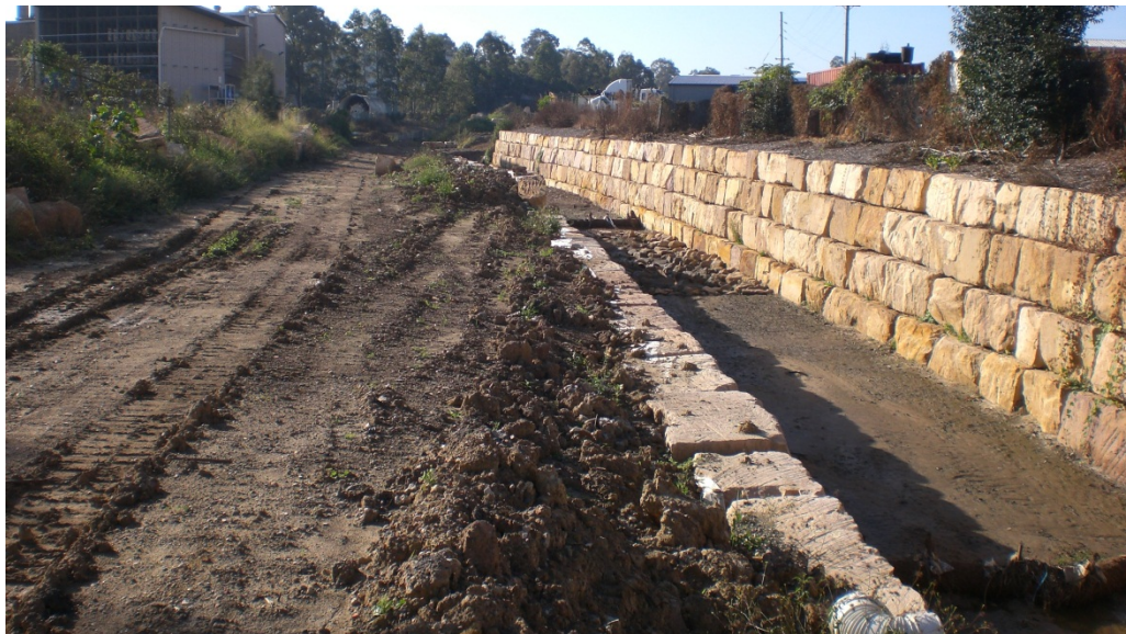
Photograph 6.4 View of recently reformed Breakfast Creek and riparian corridor outside operation boundary fence of 23-43 Tattersall Road facing east along creek.
