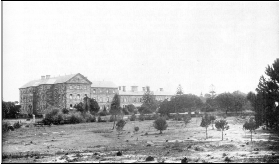
Figure 5. View east to Blackett building showing flat and bare landscape after initial tree clearance.
