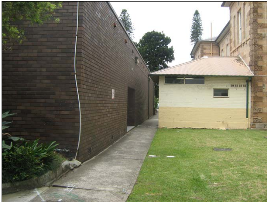
Figure 9. Open area between Oncology and Blackett Buildings showing underground services in grass and under pavement.
