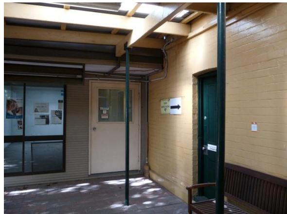
PICTURE 12 – FIRST FOOR FRONT ROOM
