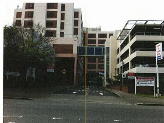
Figure 6 Existing entry to St George Hospital
