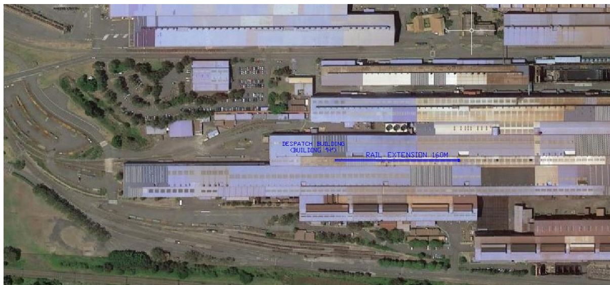
Figure 4-5 Rail Extension in Despatch Building
