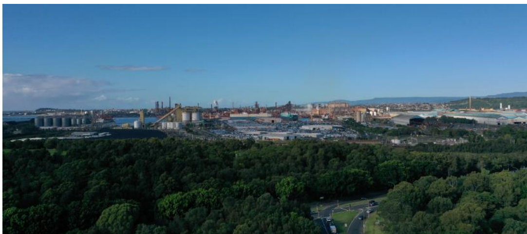
Figure 7-4 View of the large-scale Port Kembla Industrial Precinct and Port Kembla Harbour
