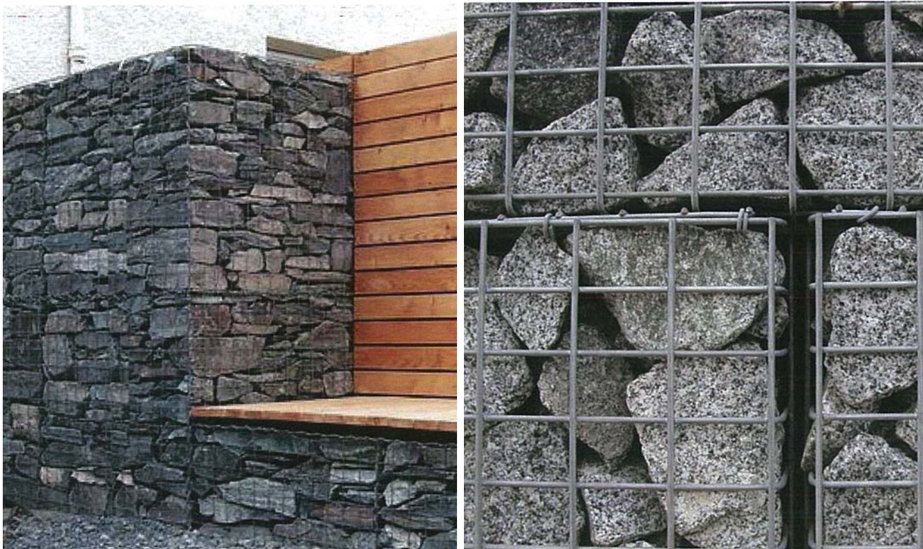
G GABION WALL
