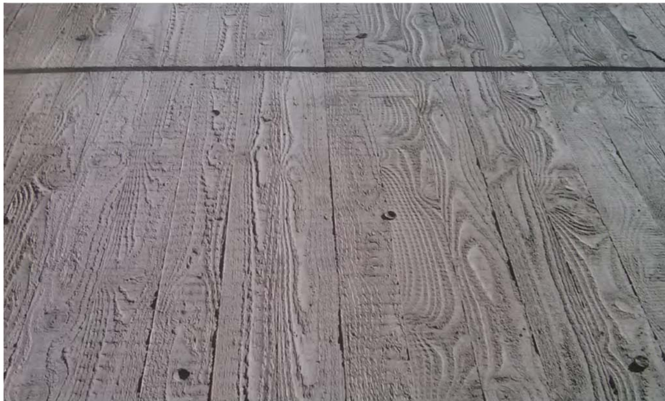
E OFF FORM CONCRETE
