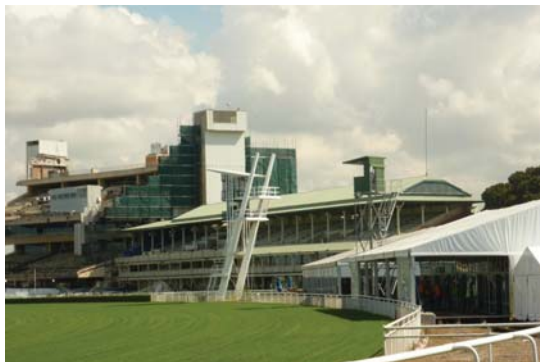
Figure 2: Photograph showing the two stewards' towers to be demolished, with the 2003 structure on the left and the post 1967 structure on the right
