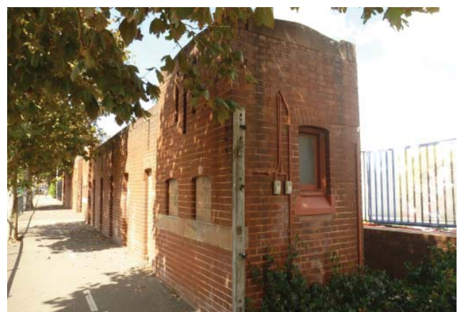
Figure 4.8 View of the former Turnstile Building, looking east, showing the bricked in openings of the former ticket booths and turnstile entrances
