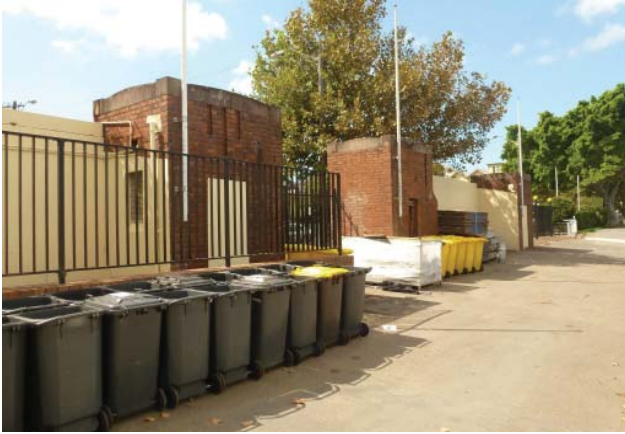
Figure 4.9 View of the former Turnstile Building showing the rear of the building has been largely demolished. The contemporary fence that is to be removed is seen in the foreground
