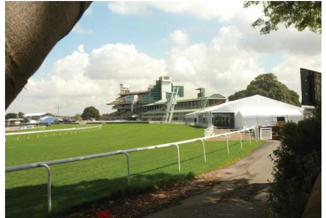
Figure 4.4 View to the subject site from the Alison Road boundary showing the Racetrack, the Oaks Marquee, the Official / Members Stand, the two Stewards Towers and the Queen Elizabeth II Stand, currently under construction
