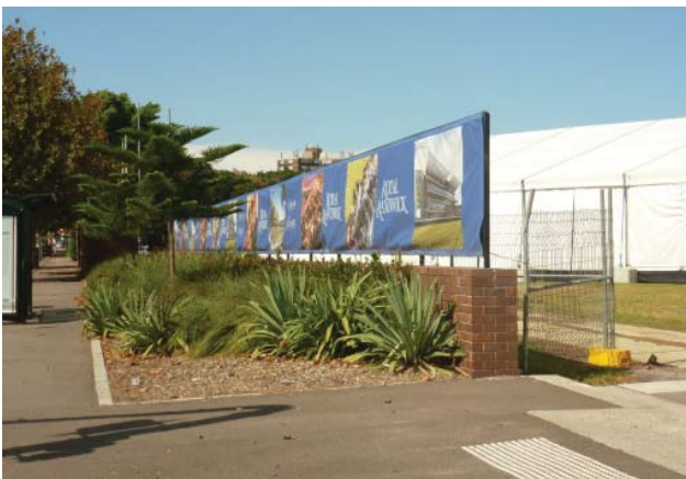
Figure 4.5 View looking east along the Alison Road frontage of the subject site showing the current boundary fence (to be demolished as part of this application) that was constructed part of the 2008 upgrade to this area
