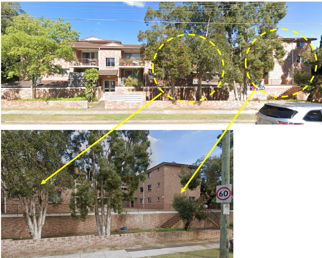
Figure 10: Northern elevation 147 Waldron Road
