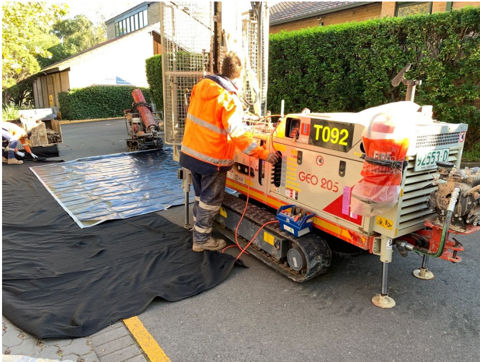
Photo 1 Borehole investigation at BH101 location
