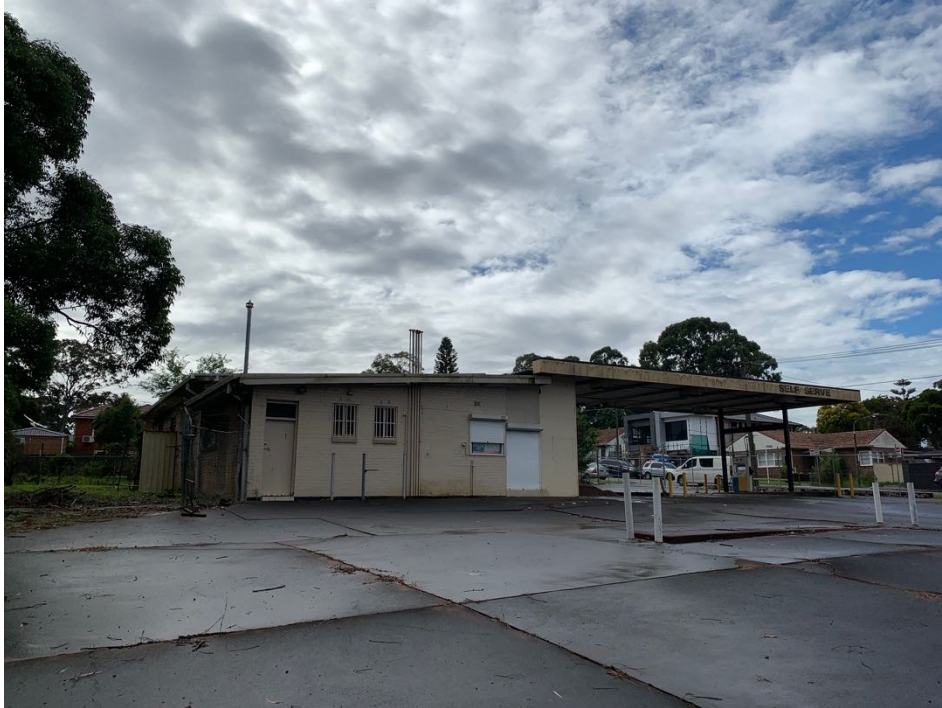
Photo 3 General overview of former service station
