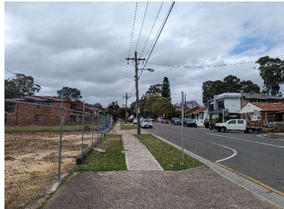
Figure 8: Streetscape view north along Campbell Hill Road
