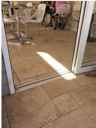
Figure 26 – Photograph of door threshold
