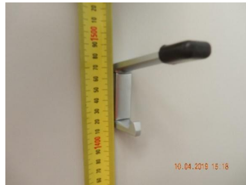
Robe Hook to be located between 1350-1500mm AFFL
