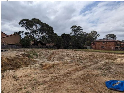
Figure 17: Vacant former service station site.
