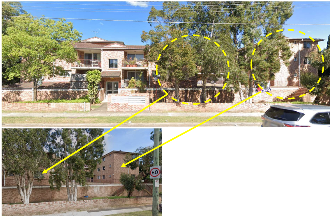
Figure 57: Northern elevation 147 Waldron Road
