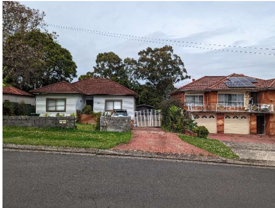
Figure 19: Dwellings on south side of Bancol Street to north of site
