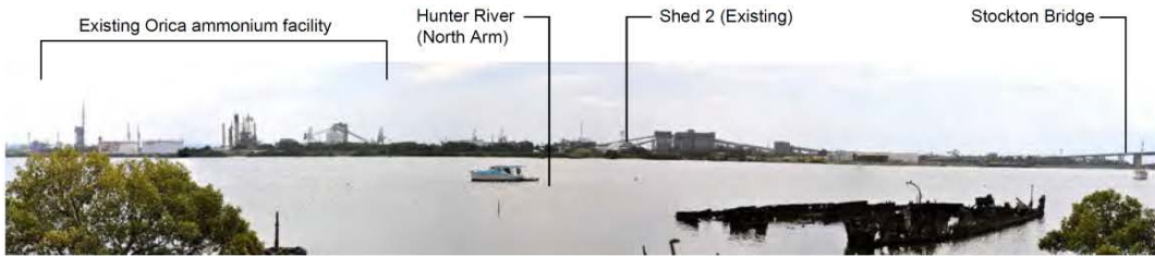
Photo Location W6 - Existing view west from Fullerton Street, Stockton
