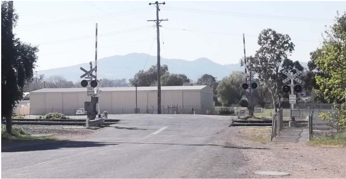
Plate 11 Nowland Street Railway Level Crossing
