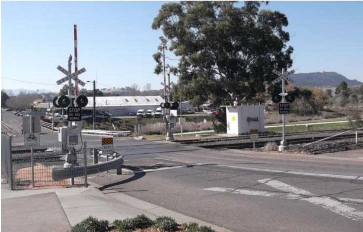
Plate 10 Henry Street Railway Level Crossing
