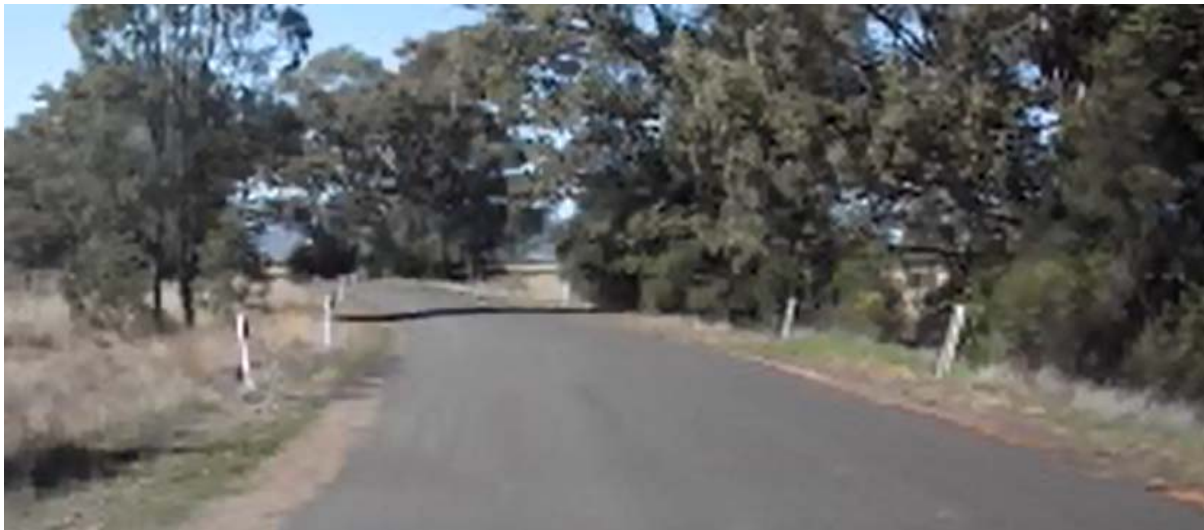
Plate 8 Culvert Crossing on Bulunbulun Road
