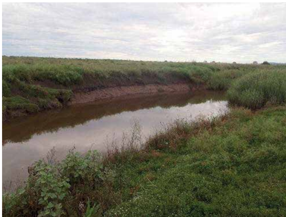
Figure 3-9 Evidence of Bank Failure is Common Along the Lower Reach of Native Dog Gully
