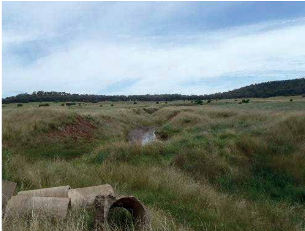
Figure 3-5 Upstream View of a Channelised Fill Section of an Unnamed Western Tributary of Watermark Gully
