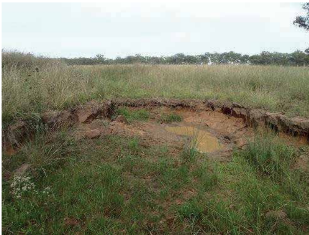
Figure 3-8 Upstream View of a Headcut on Watermark Gully
