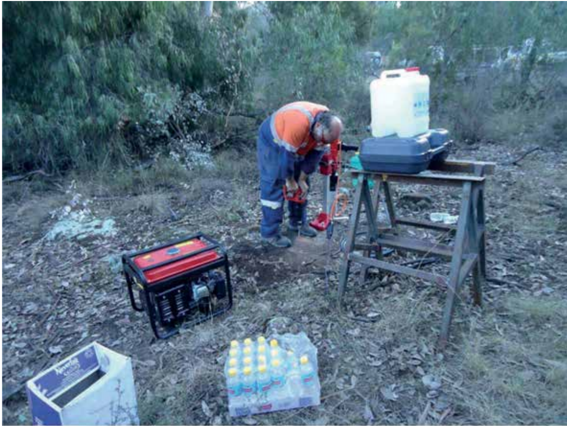
Photo 20: Setting up of the drill site at WM-GG3-12.
