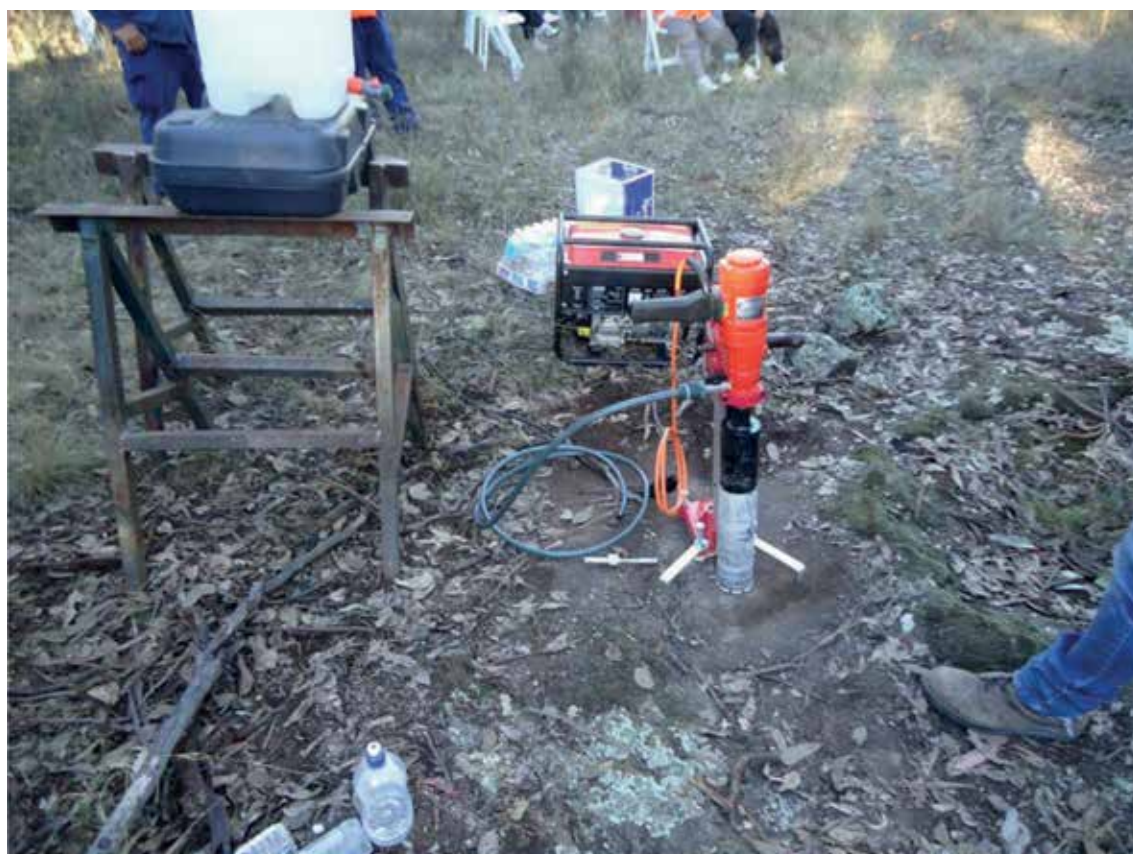
Photo 19: View of the drill setup to core the bedrock.
