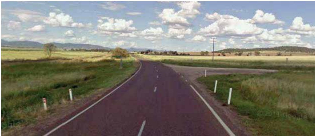
Plate 2 Looking southbound on Kamilaroi Highway towards The Dip Road.
