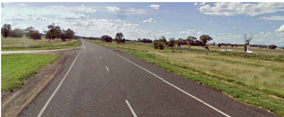
Plate 3 Looking northbound on Kamilaroi Highway towards Court Lane.
