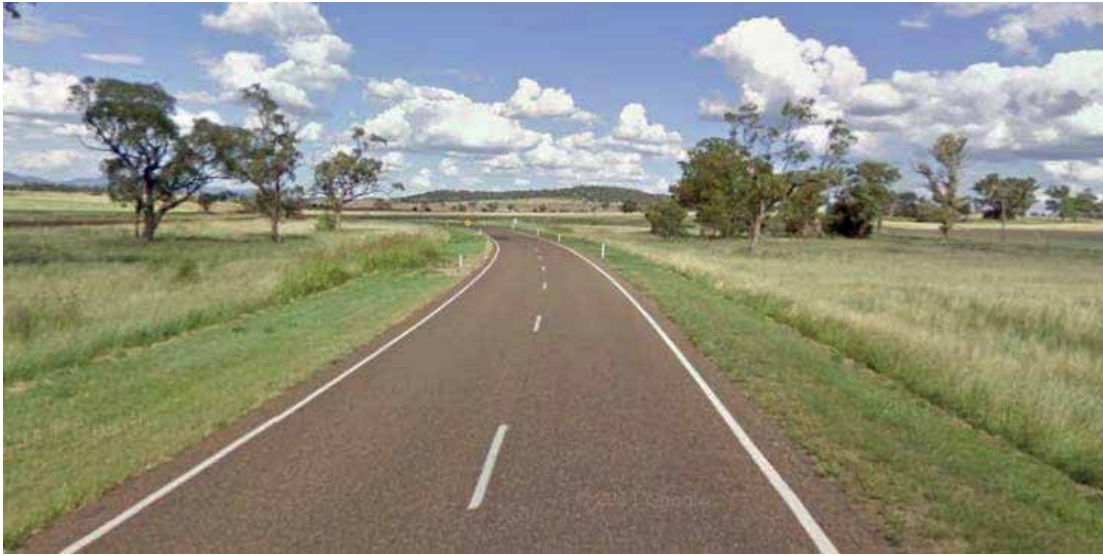
Plate 1 Looking south on the Kamilaroi Highway towards The Dip Road
