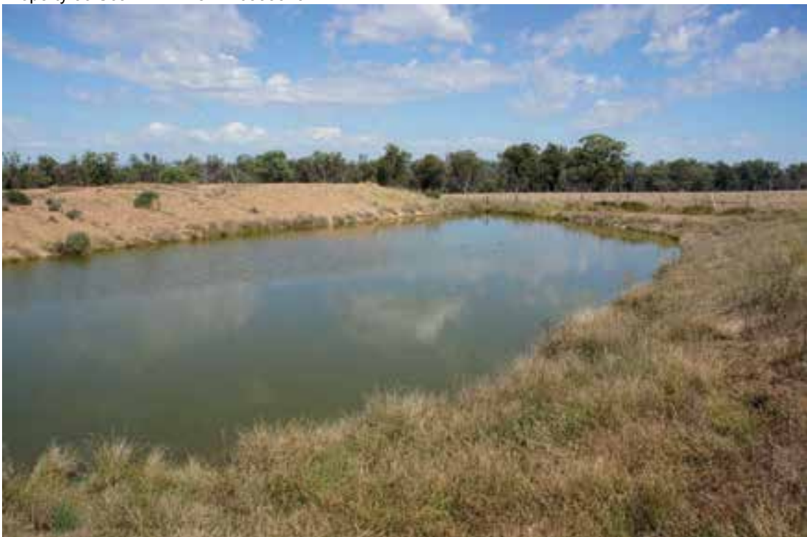
Property 19 Spring Fed Dam E 243227 N 6535286
