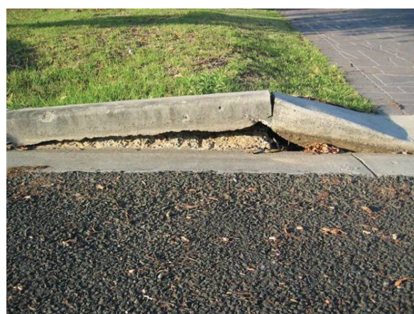
Fig. 5.4 Cracking and Buckling of Kerb in the Southern Coalfields
