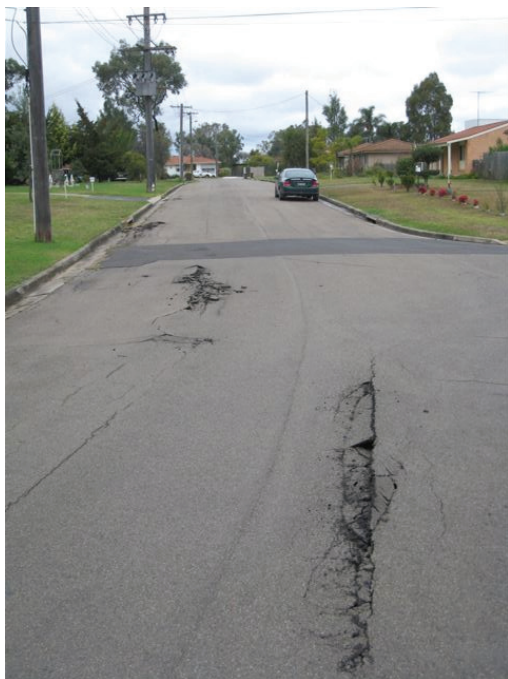
Fig. 5.3 Cracking and Bump at Roundabout in the Southern Coalfields
