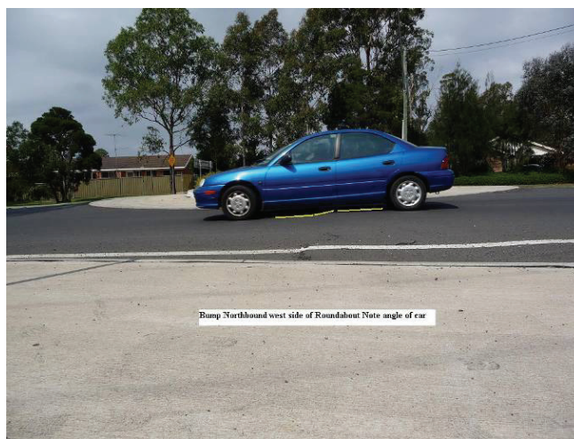
Fig. 5.3 Cracking and Bump at Roundabout in the Southern Coalfields
