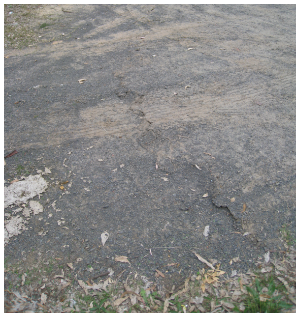
Fig. 4.10 Example of Surface Compression Buckling Observed in a Pavement
