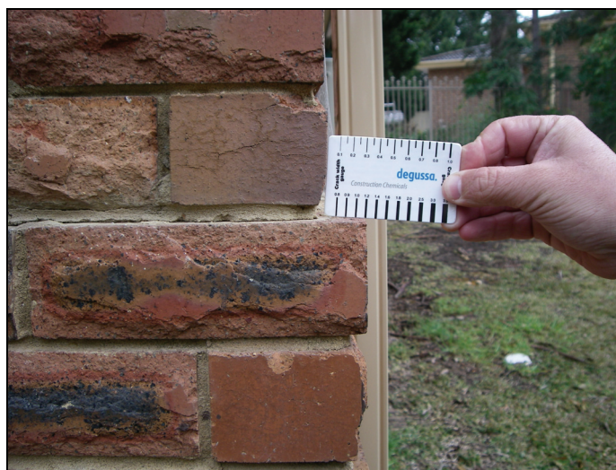
Fig. C.1 Example of slippage on damp proof course
