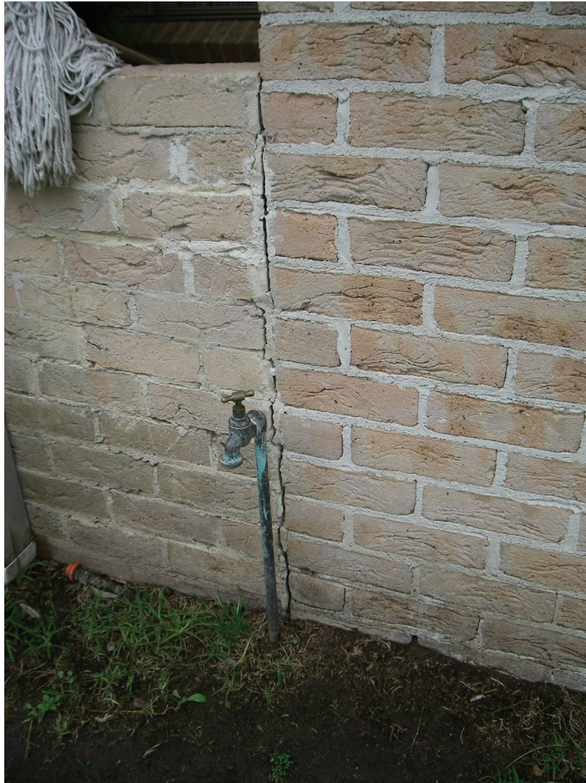
Fig. C.2 Example of crack in mortar only
