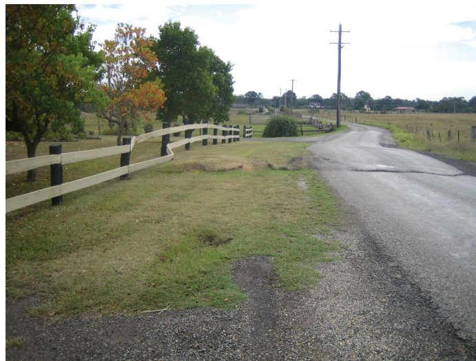
Fig. 4.9 Example of Surface Compression Humping along Outcropping of a Low Angle Thrust Fault in the Southern Coalfield
