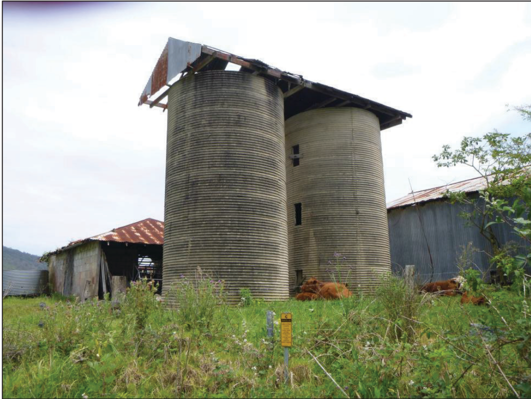
Plate 21: Keegan's silo (Table 3, Item O), within the Subsistence Impact Limit. The concrete veneer shed can be seen in the background as part of a larger shed complex.
