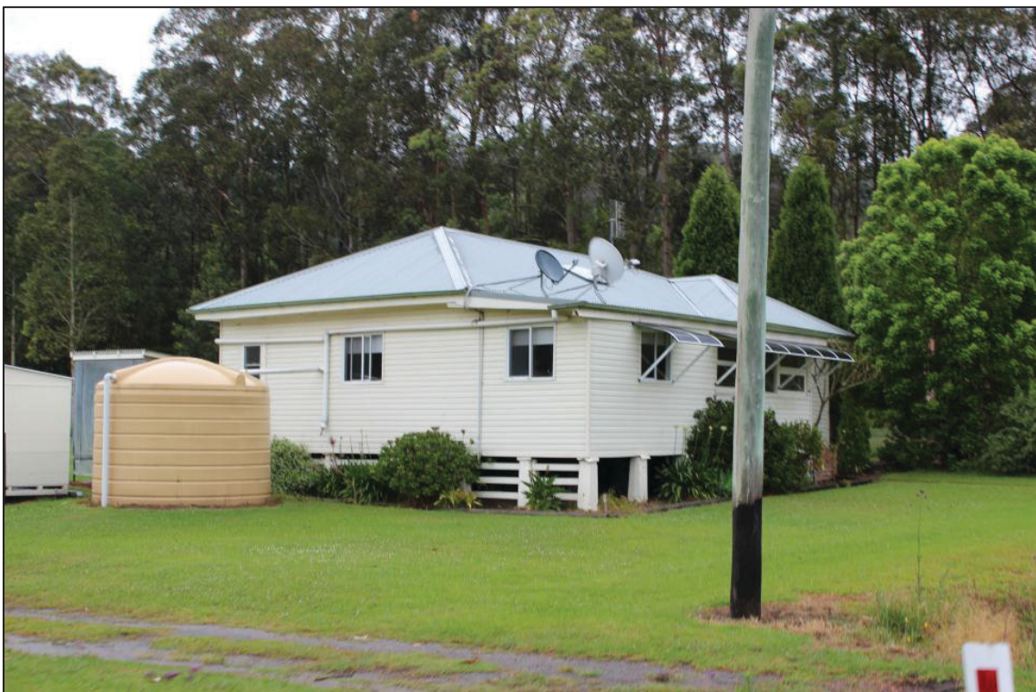
Plate 15: This view of Item J was taken from Little Jilliby Road ( Table 3 ). As with items G, S, and R, the item has not been previously assessed beyond having potential heritage significance, and no new significance is attributed to the item here. Source: Hansen Bailey.
