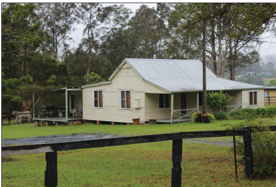
Plate 24: This cottage (Table 3; Item S) is similar to others in the area and was not assessed as reaching a local level of significance. Source: Hansen Bailey.
