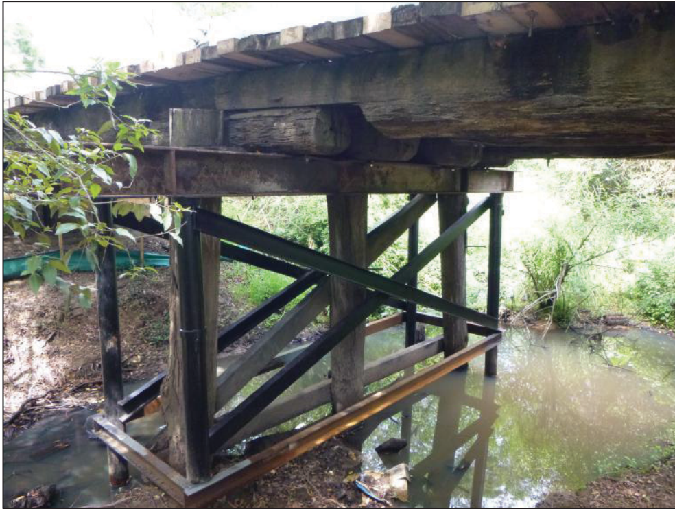
Plate 18: Steel girders have somewhat compromised the aesthetic value of the bridge, but a large portion of the original elements are intact.
