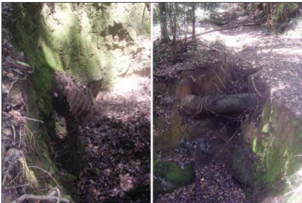
Plate 12: WSF-HS1: Different phases of culverts beneath the forestry road along Little Jilliby Jilliby Creek. On the left is the older form of drain made from tin, while a concrete drain to right suggests the road was re-engineered at some point and new drainage features installed.
