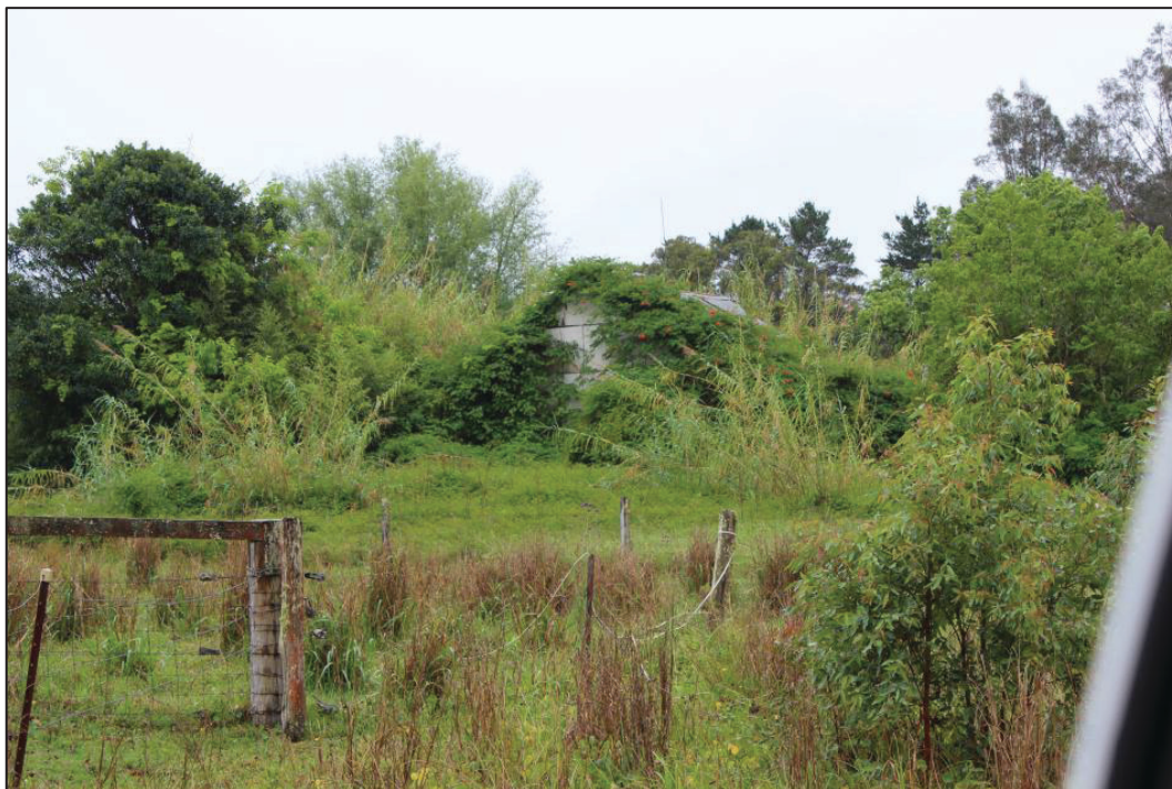
Plate 23: This barn or cottage ( Table 3 , Item R) was difficult to assess due to the heavy overgrowth. This very factor diminishes the potential heritage value of the item though. Source: Hansen Bailey
