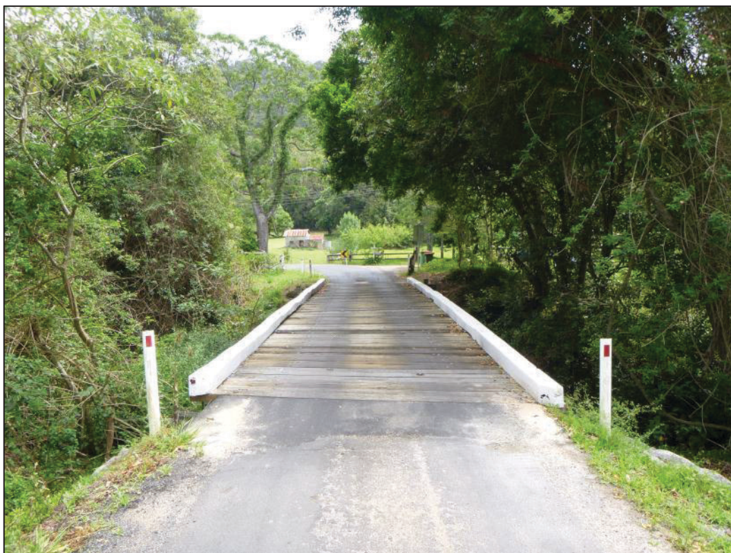
Plate 17: View north along the bridge over Little Jilliby Road ( Table 3 ; Item M). This assessment suggests the bridge has a local level of heritage significance.
