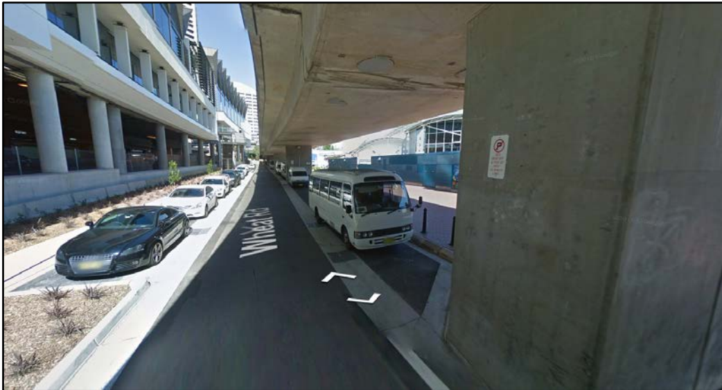
Figure 2 | Current (proposed) layout of Wheat Road as viewed looking south (Source: Google Maps)
