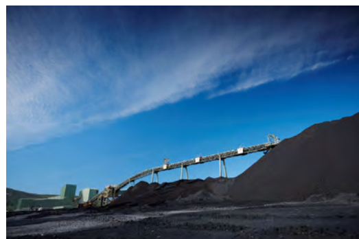
Plate 1: SMC CHPP and Product Coal Stockpile.
