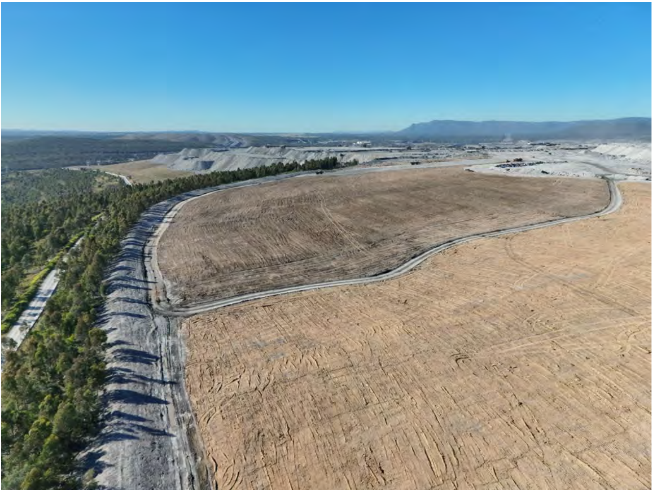
Photo 8.2 Topsoil Spread at the Northern Extension 2025
