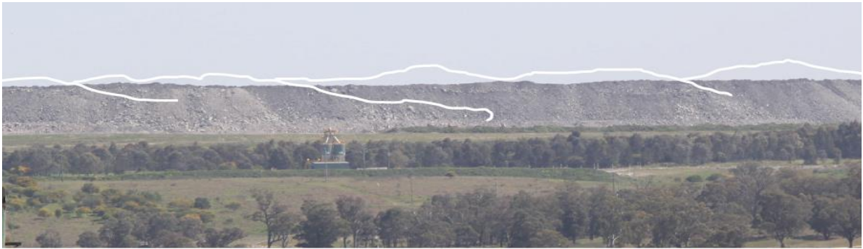
Figure 3.13 | Example of a typical bund with suggested modifications to profile, considered in Workshop C
