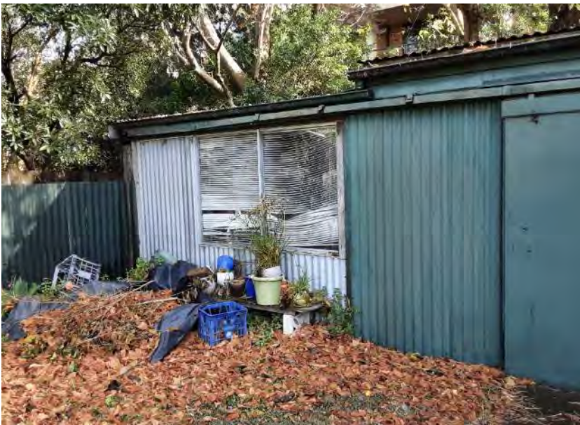
Photo 19 Domestic shed within Lot 30 DP4785, facing north-west
