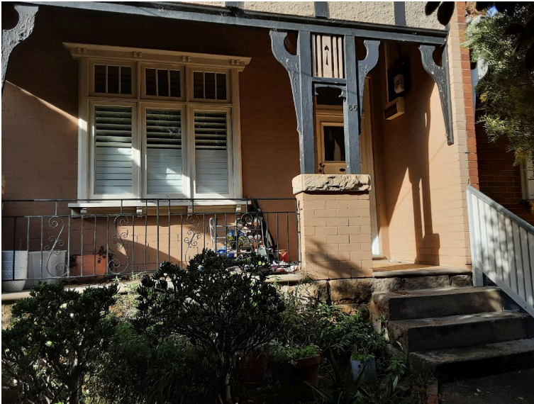
Photo 18 Brick residence [14] constructed c.1910 at 65 Gerard Street
