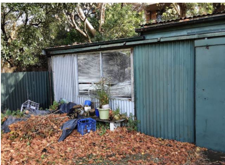
Photo 13 Shed located at the rear of 50 Parraween Street
