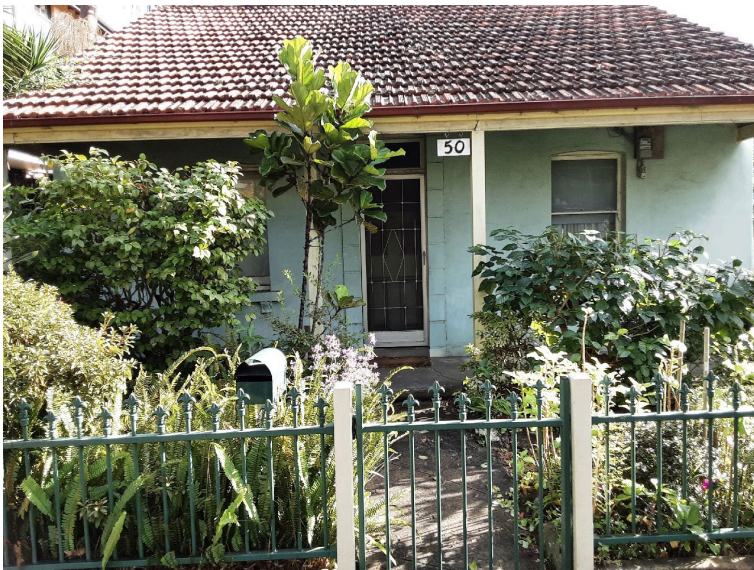
Photo 10 The original pre 1890 brick residence [1] at 50 Parraween Street
