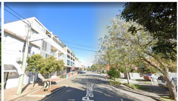
Photo B: Parraween streetscape south east view
