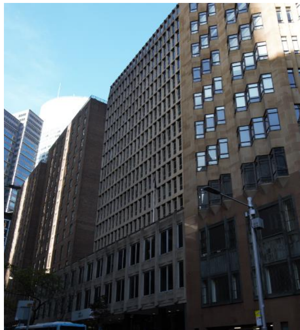
Figure 8 – View of the subject property facing north east. The set back of the tower is visible, and the projection of the concrete columns is evident.
