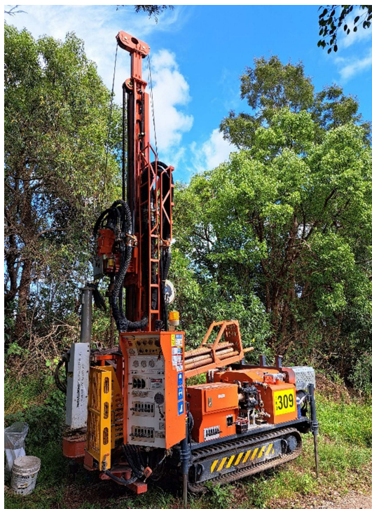
Photo 14 - Hanjin DB8 drill rig, 24 January 2023
