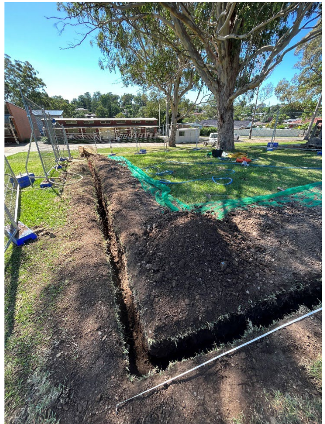
Figure 7: Northern portion of trench following excavation
