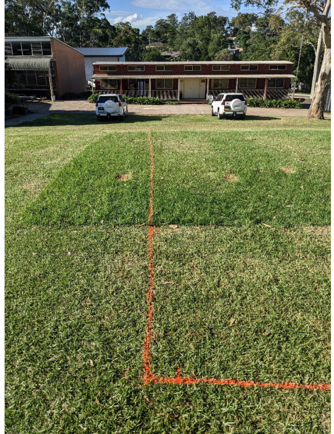
Figure 5: Set-out for northern portion of trench.
