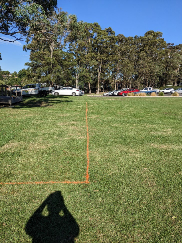
Figure 4: Set-out for eastern portion of trench
