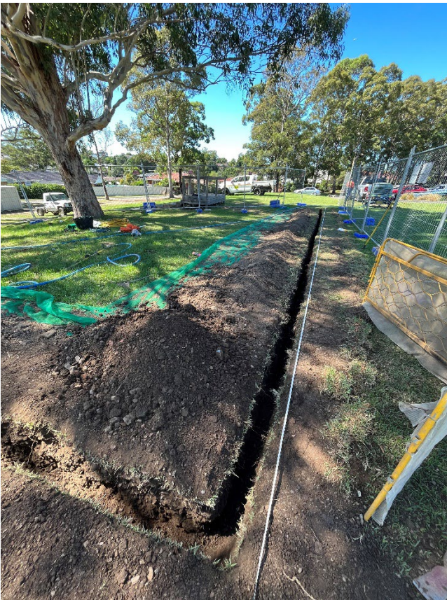
Figure 6: Eastern portion of trench following excavation
