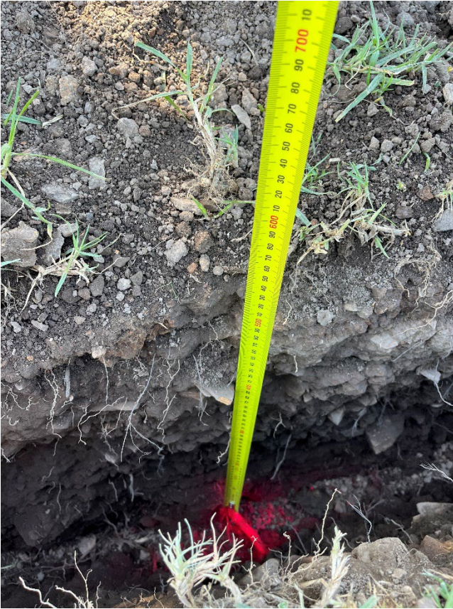
Figure 12: Excavation depth achieved
