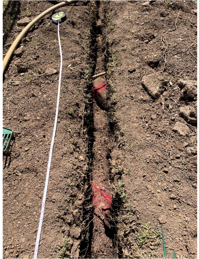
Figure 9: Roots 5 & 6 within the northern portion of the trench
