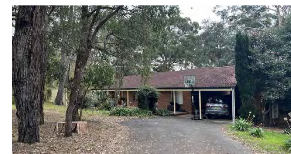
HAWKHURST COTTAGE - TO BE DEMOLISHED
