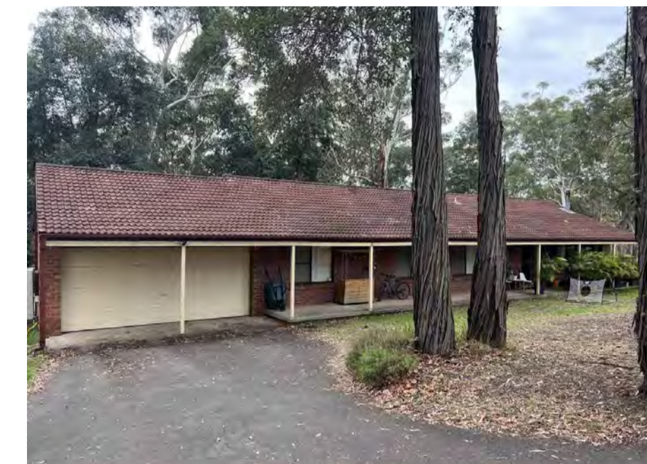
ANLISS COTTAGE - TO BE DEMOLISHED
