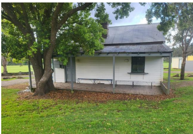
Figure 120 Early 20 th century Cottage proposed for demolition
