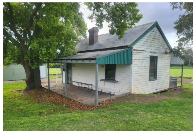
Figure 121 – Early 20 th century Cottage proposed for demolition
