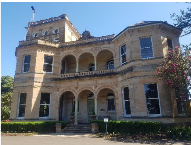
Figure 40 - Two projecting hexagonal bays with double-hung windows are located on either side of a recessed entrance with a triple-arched porch
