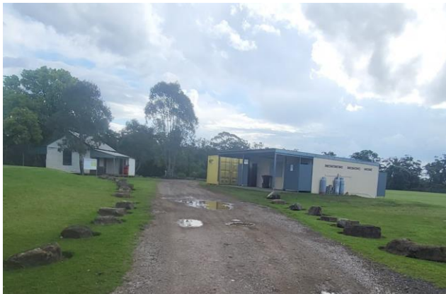
Figure 118 View west along Massie Road showing the amenities block (right) and early cottage (left)
