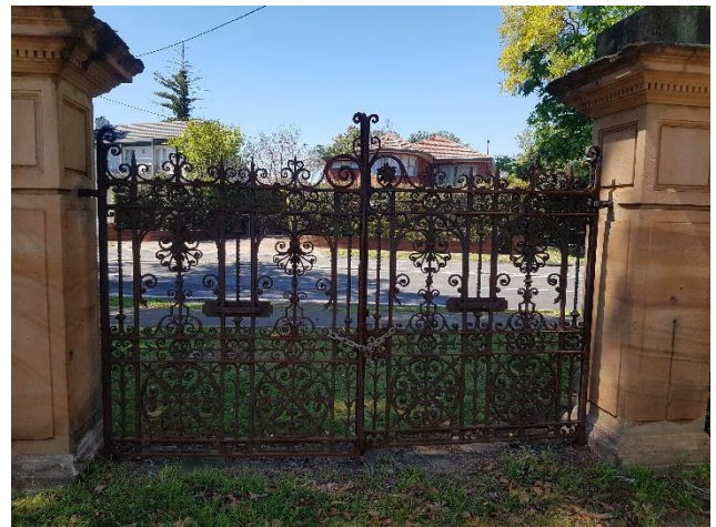
Figure 50 – A wrought iron entrance gate with sandstone posts opens to Pennant Hills Road
