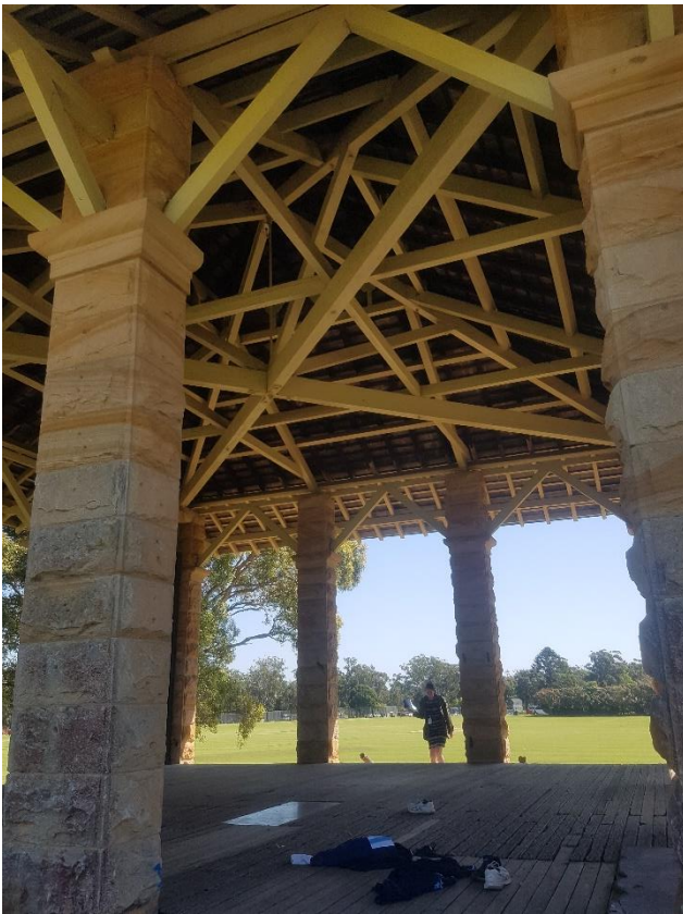
Figure 53 View of the roof structure.
