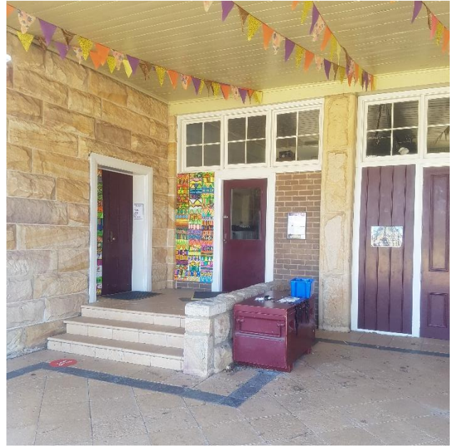
Figure 47 - The former stable spaces have been infilled with brick walls, timber doors and windows and the ground paved for the building's current use as the Music Centre.
