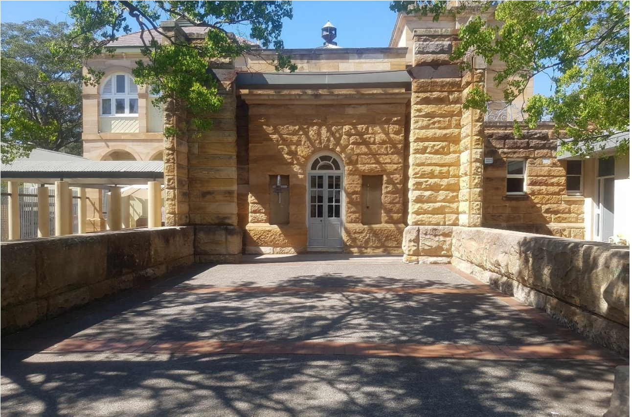
Figure 42 - The north-eastern elevation of Gowan Brae has a rough-textured sandstone block façade
