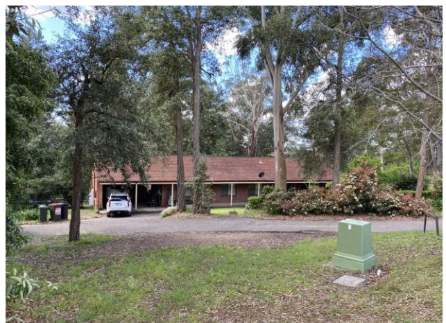
Figure 124 – View of the c.1980s Angliss cottage proposed to be demolished
