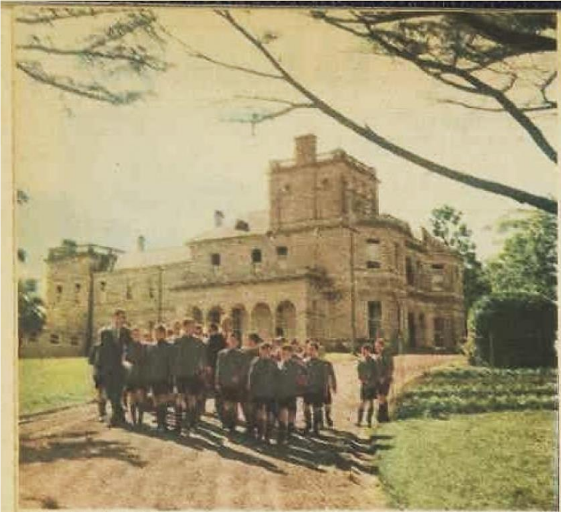
GOWAN BRAE, Victorian mansion on the property which will be the site of the new King's School, is now used as a preparatory school for 75 day-boys and 75 boarders. It was originally the home of Scottish philanthropist-trader Sir James Burns.
