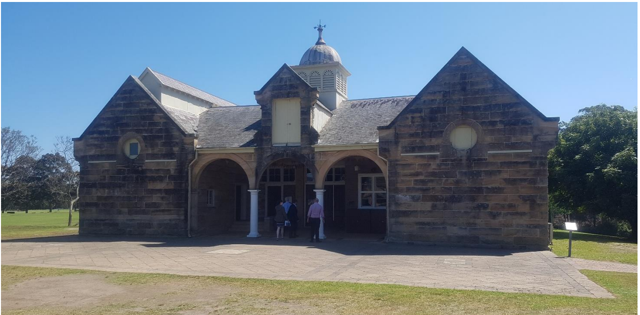
Figure 45 - Two bays with pitched roofs and ocular windows sit on either side of a recessed entrance which sits behind three arches supported on Doric columns.
