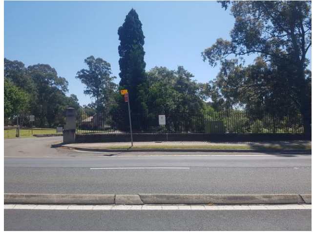
Figure 74 View of the iron palisade fence and stone hob
