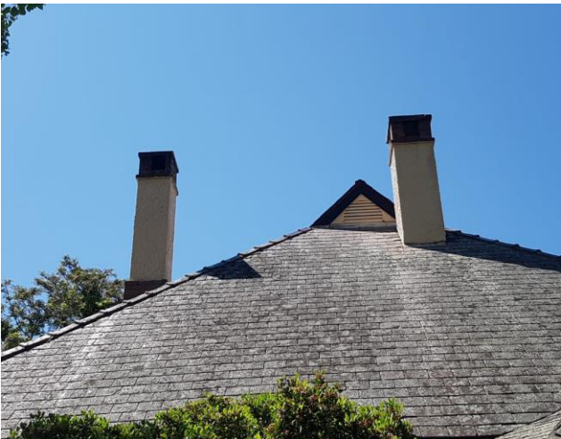
Figure 61 – Slate roof of “The Cedars” with Dutch gable and two chimneys
