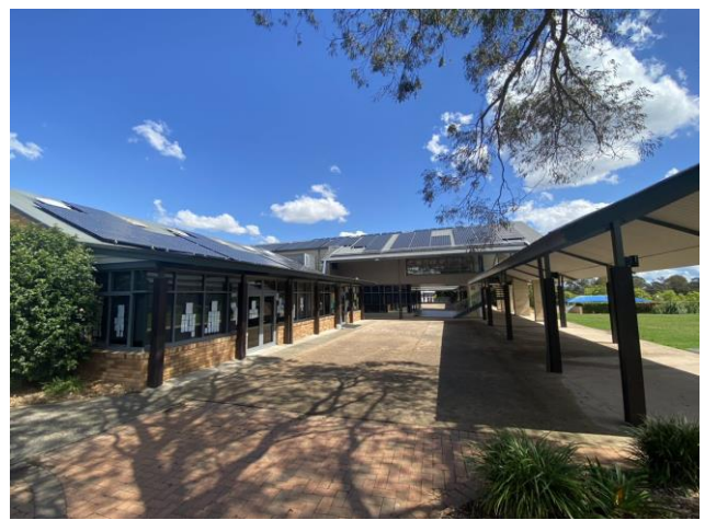
Figure 30 – Rear of the Preparatory School
