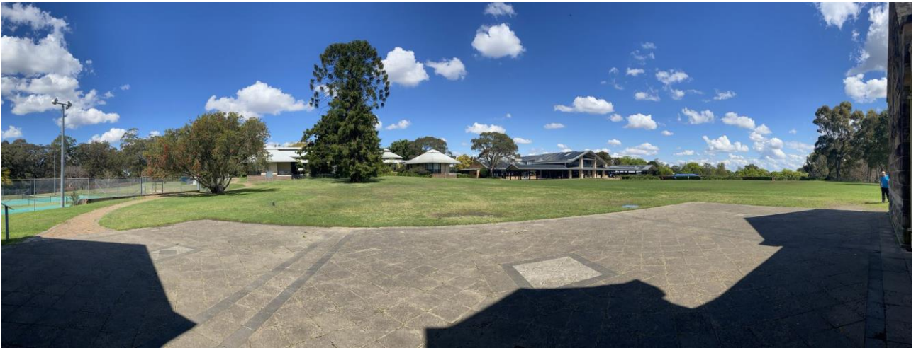
Figure 82 View towards the rear of Gowan Brae and the Prep school, and showing the general grounds and setting including mature Norfolk Island tree plantings, fields and part view of tennis courts
