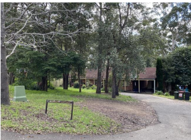
Figure 123 View of the c.1980s Hawkhurst cottage proposed to be demolished
