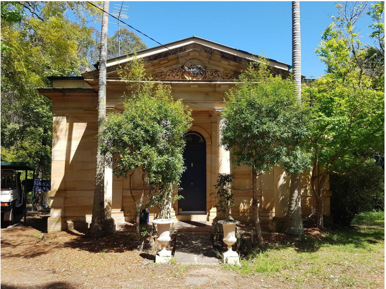
Figure 48 - The Gatehouse is a fine-chiselled sandstone Classical structure with large decorative pediment supported on four columns
