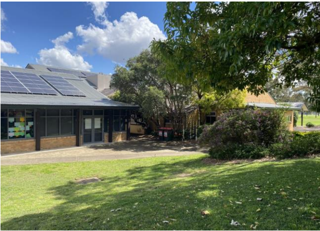
Figure 27 - The Prep Administration Building (left) and Dalleywater Centre (right)
