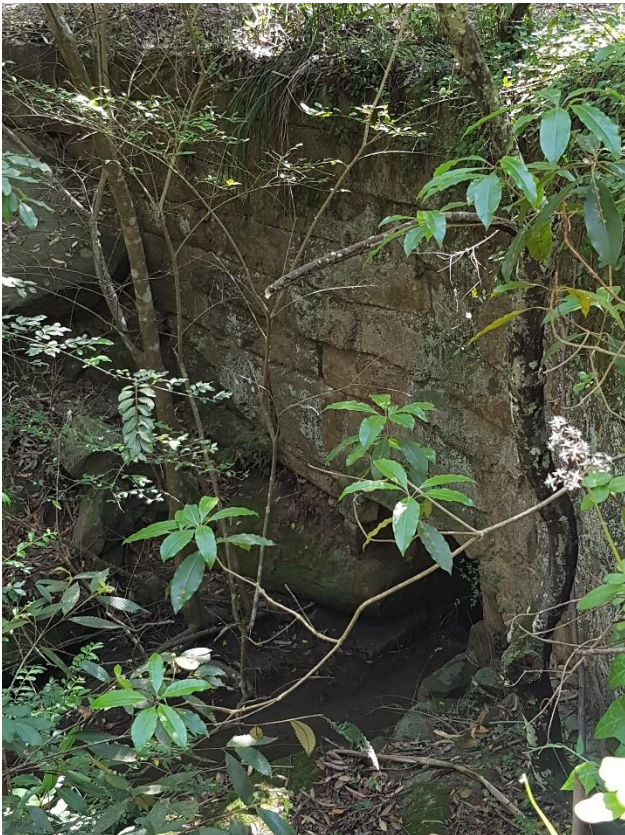
Figure 71 – Detail of the sandstone constructed horseshoe dam
