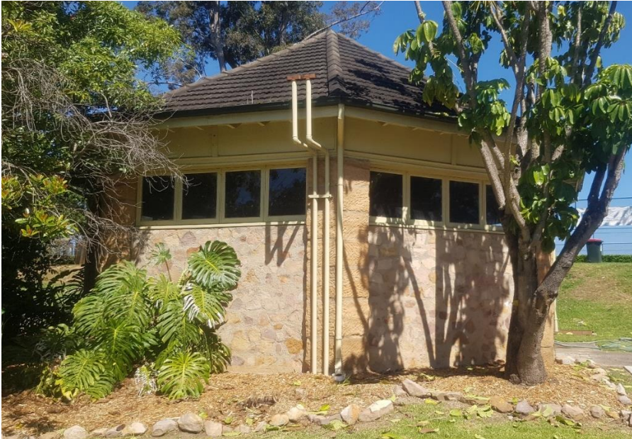
Figure 65 - Approximately 300 metres north of Gowan Brae House is the former Rotunda, which originally consisted of a pitched roof supported on 5 rough-cut sandstone columns
