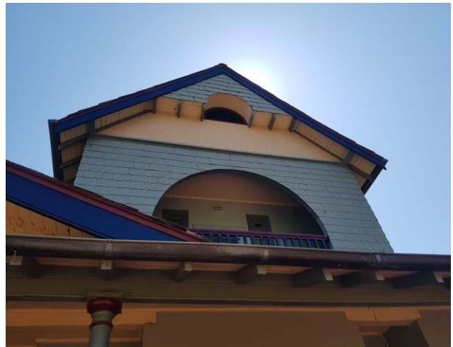
Figure 62 – A large dormer with shingled façade encloses a recessed balcony with arched opening
