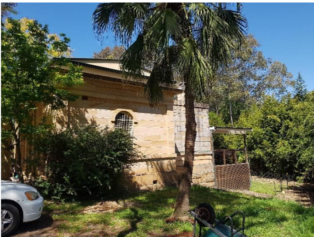
Figure 49 - A timber addition is located at the rear of the Gatehouse
