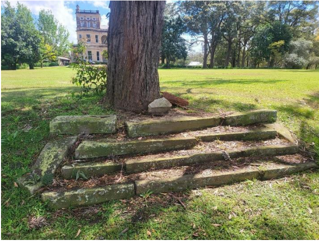
Figure 53 – Sandstone steps to the south-east of Gowan Brae, which are partially covered by the turfing of the area.
