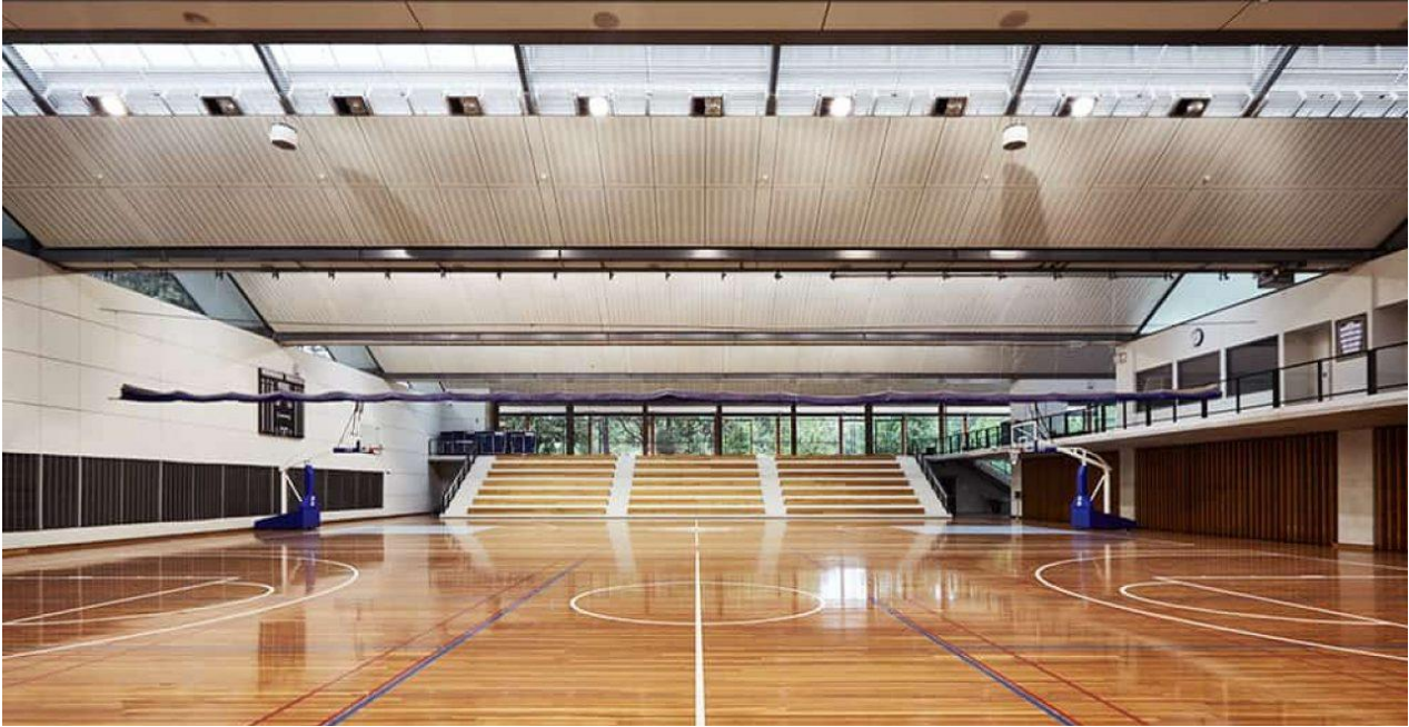
Figure 63 – Interior of the Senior School Sports Centre, showing the sub-surface level of basketball courts, relative to the ground level.
