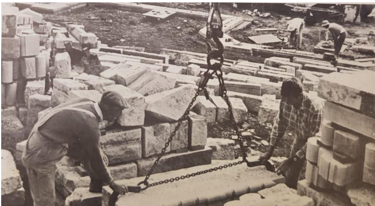
Figure 43 – Skilled craftsmen rebuild the Chapel
