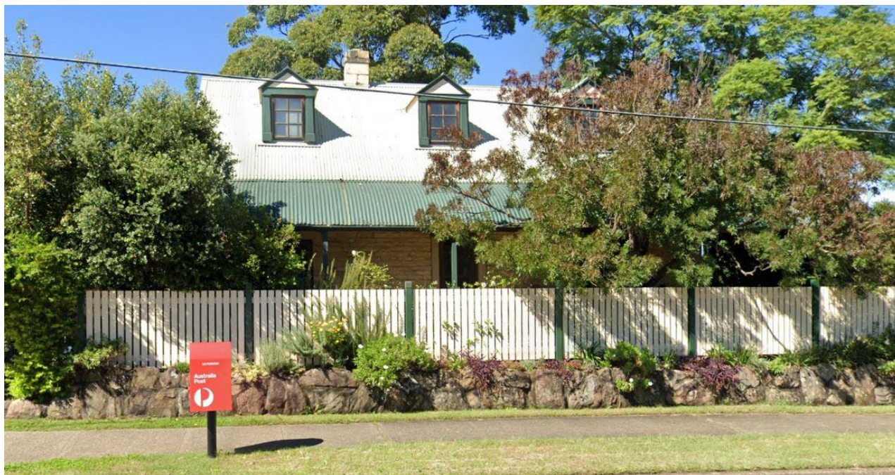
Figure 23 – Front elevation of 224 North Rock Road, North Rocks 2151 "Rockcliff". Note the building materials, which include a sandstone cottage and retaining wall, timber detailing and picket fence, and tin roofing.
