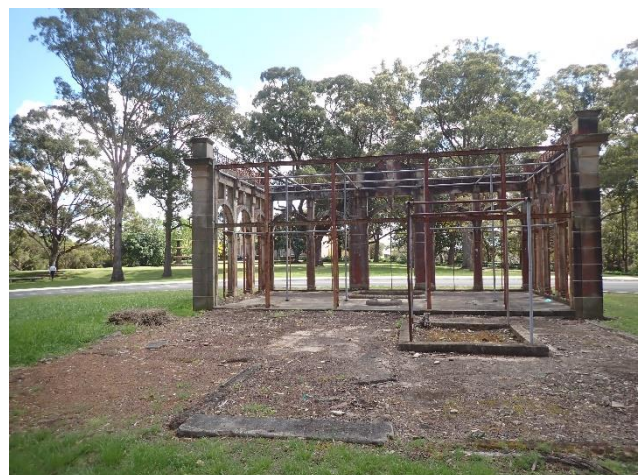
Figure 58 – Potential flooring identified as exposed to the south of the Aviary.
