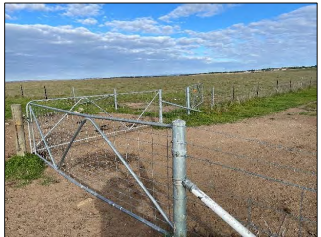
Plate 6: Agricultural infrastructure within the Project Area includes fencing and gates.
