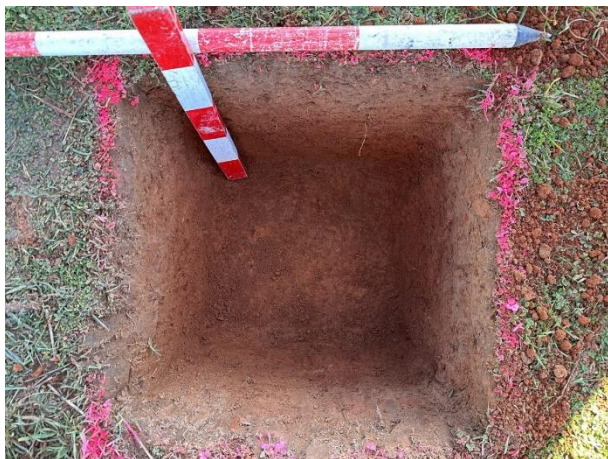
End of excavation
