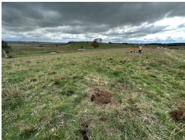
Backfilled trench, facing north.
