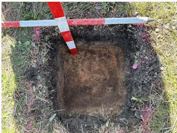
End of excavation
