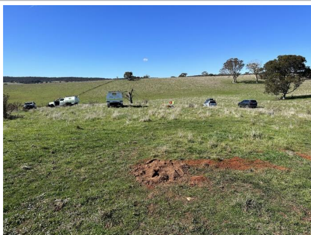
Backfilled trench, view east
