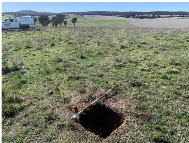
Pre-excavation, view north-east
