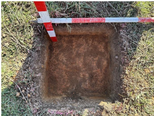
End of excavation
